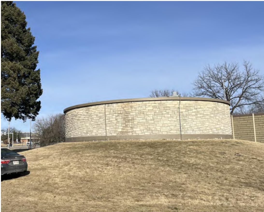
Existing Reservoir to be removed and replaced.
