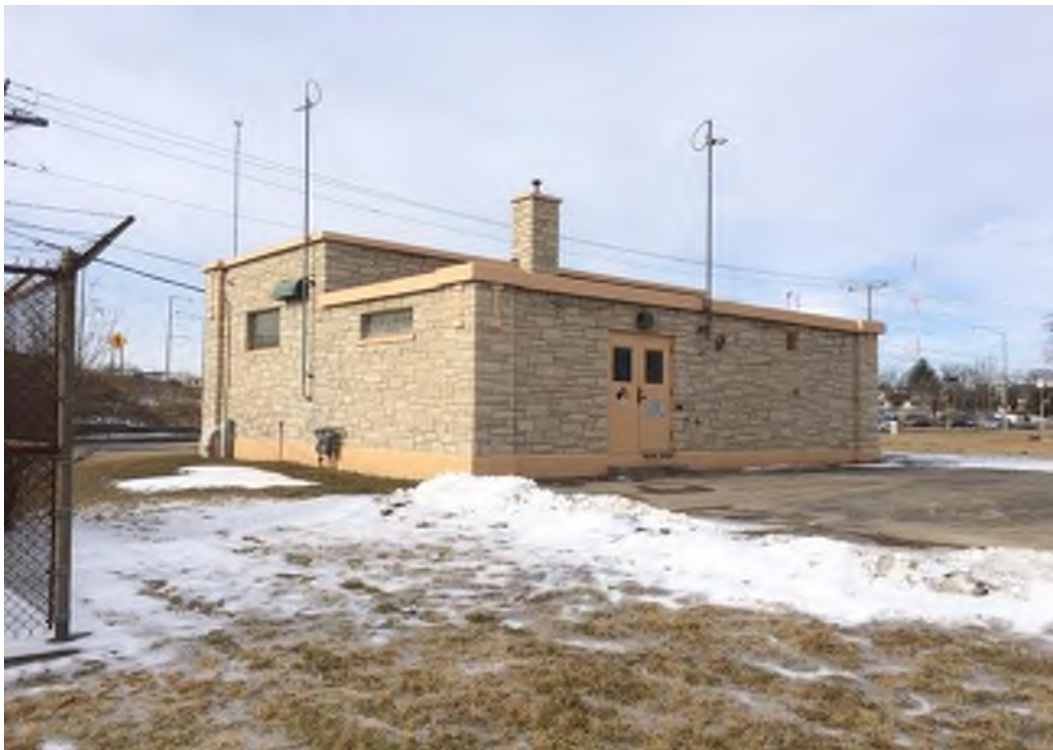
The rear of the existing Wellhouse.
