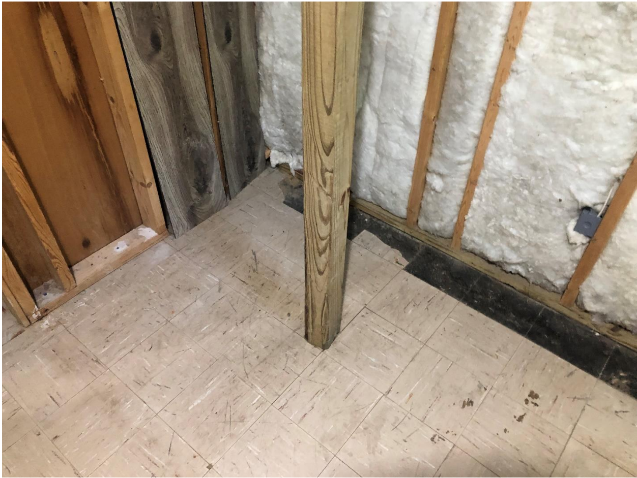
Image showing lack of attachment and lack of foundation at the base of wood columns.
