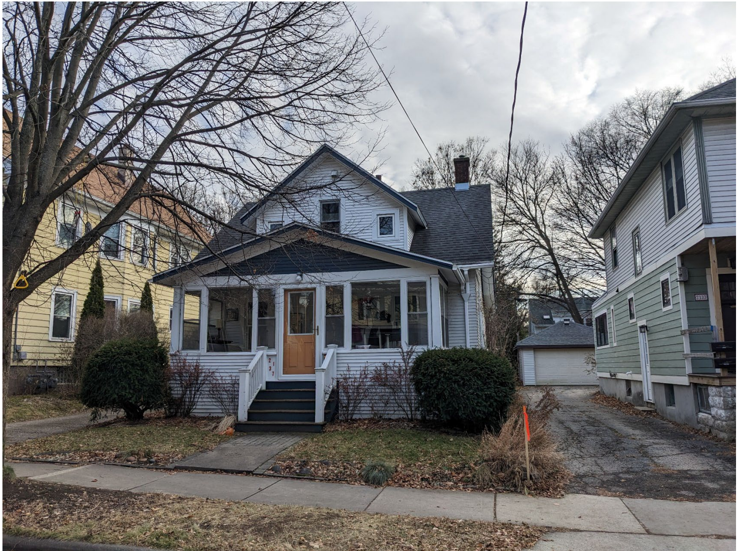
FRONT NORTH ELEVATION FROM STREET
