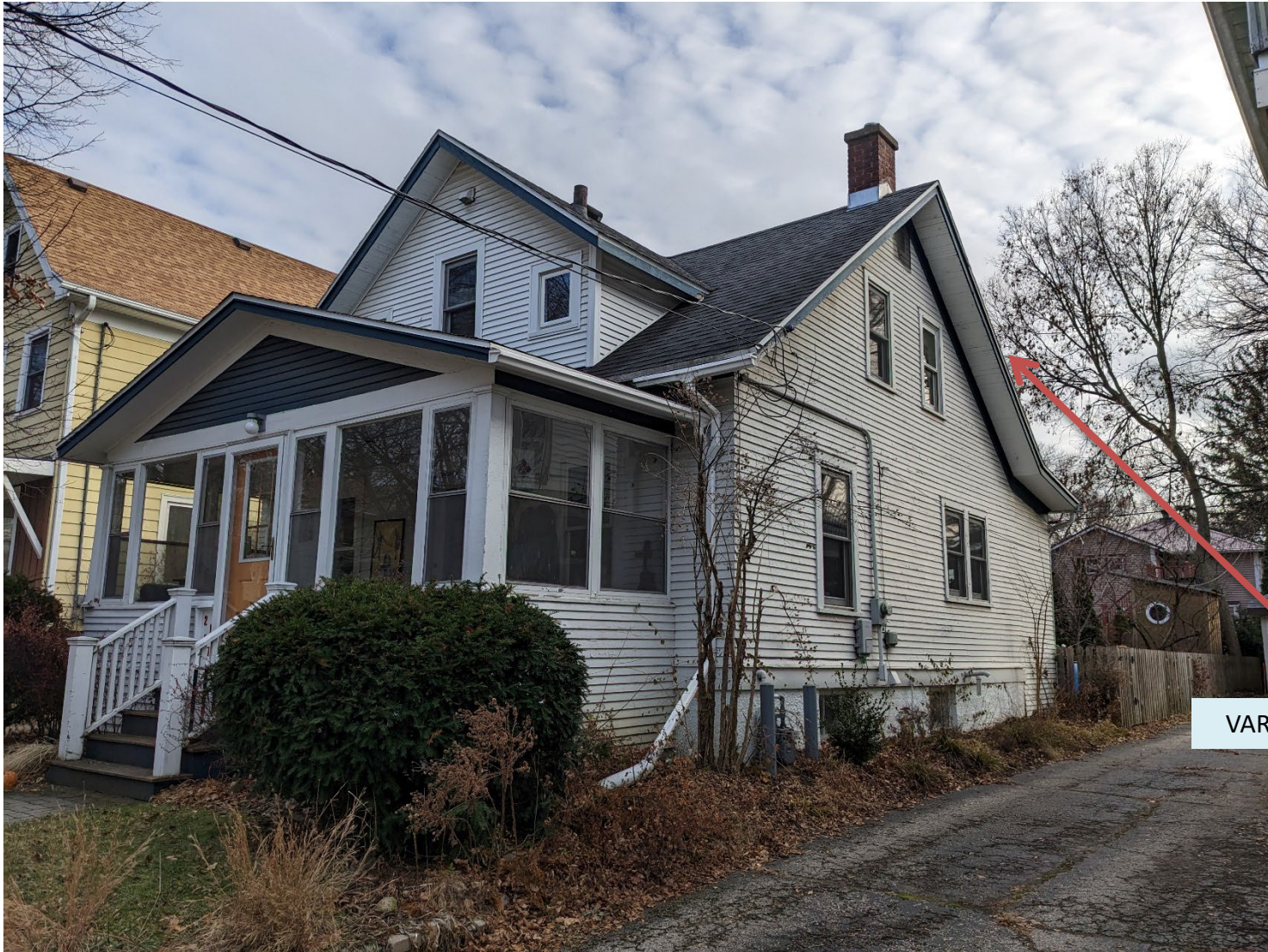
FRONT NORTH ELEVATION AND WEST SIDE ELEVATION FROM STREET
