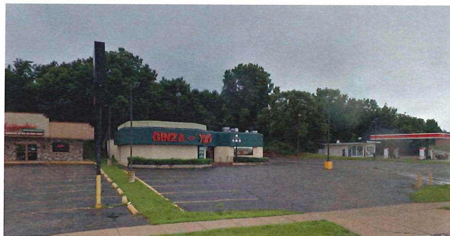
BOTH ADJACENT BUILDINGS
