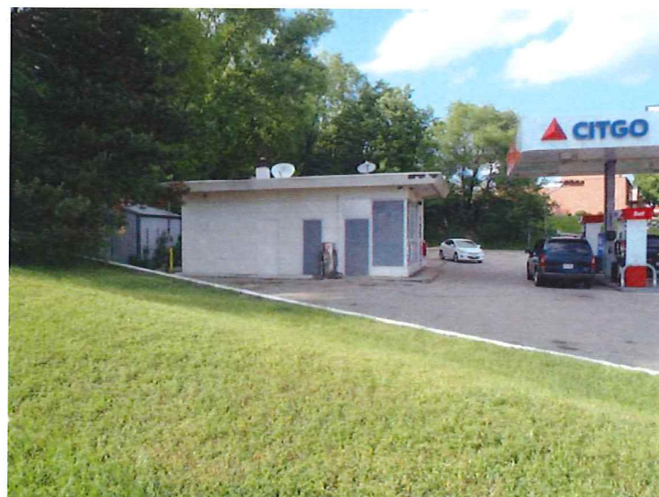
ADJACENT GAS STATION TO EAST
