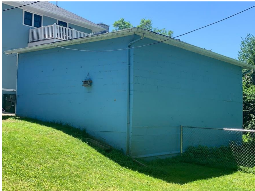
Existing garage (North)
