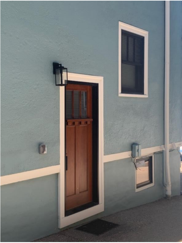
Main House side entry door
