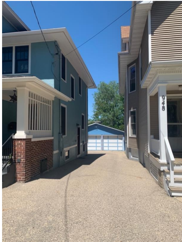
Shared driveway to garage
