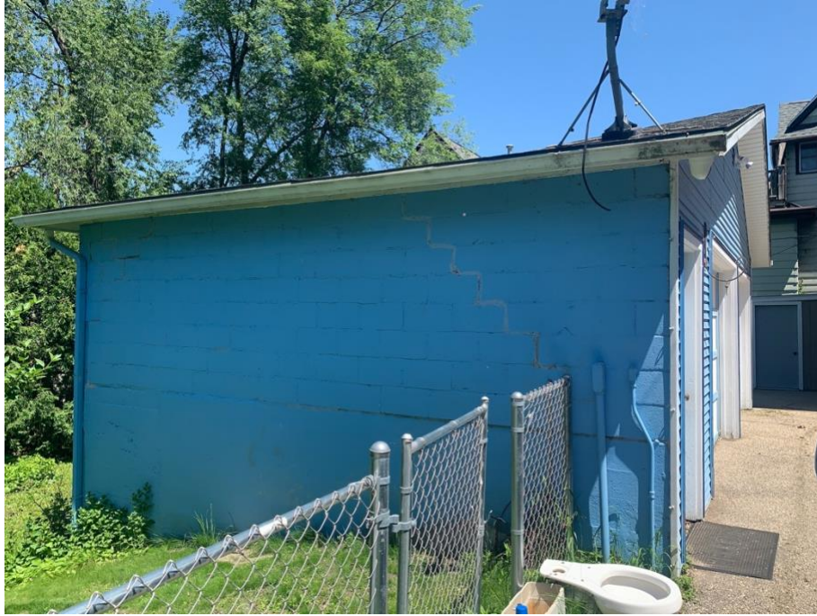
Existing garage (South)
