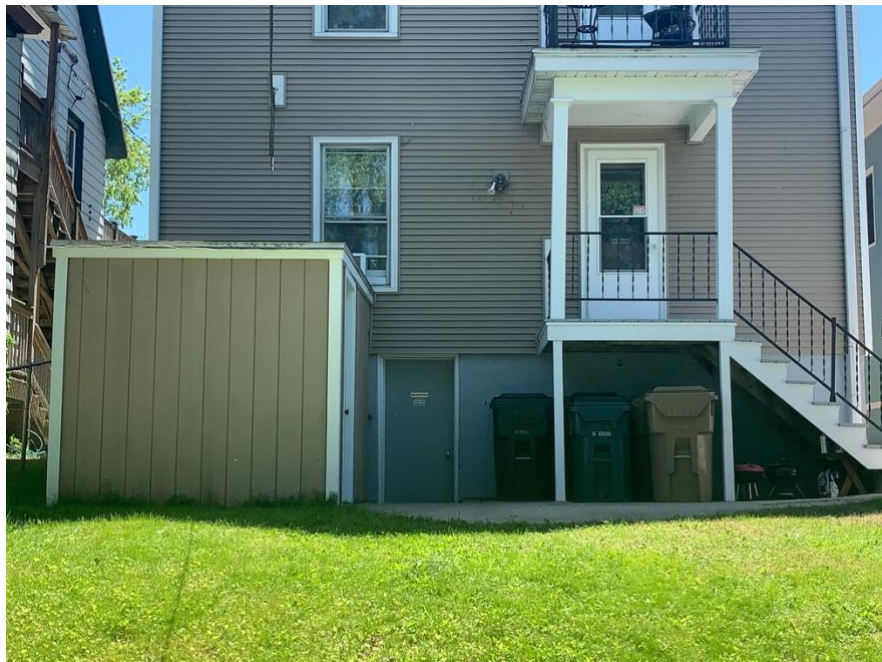
Rear view of 948 Jenifer house
