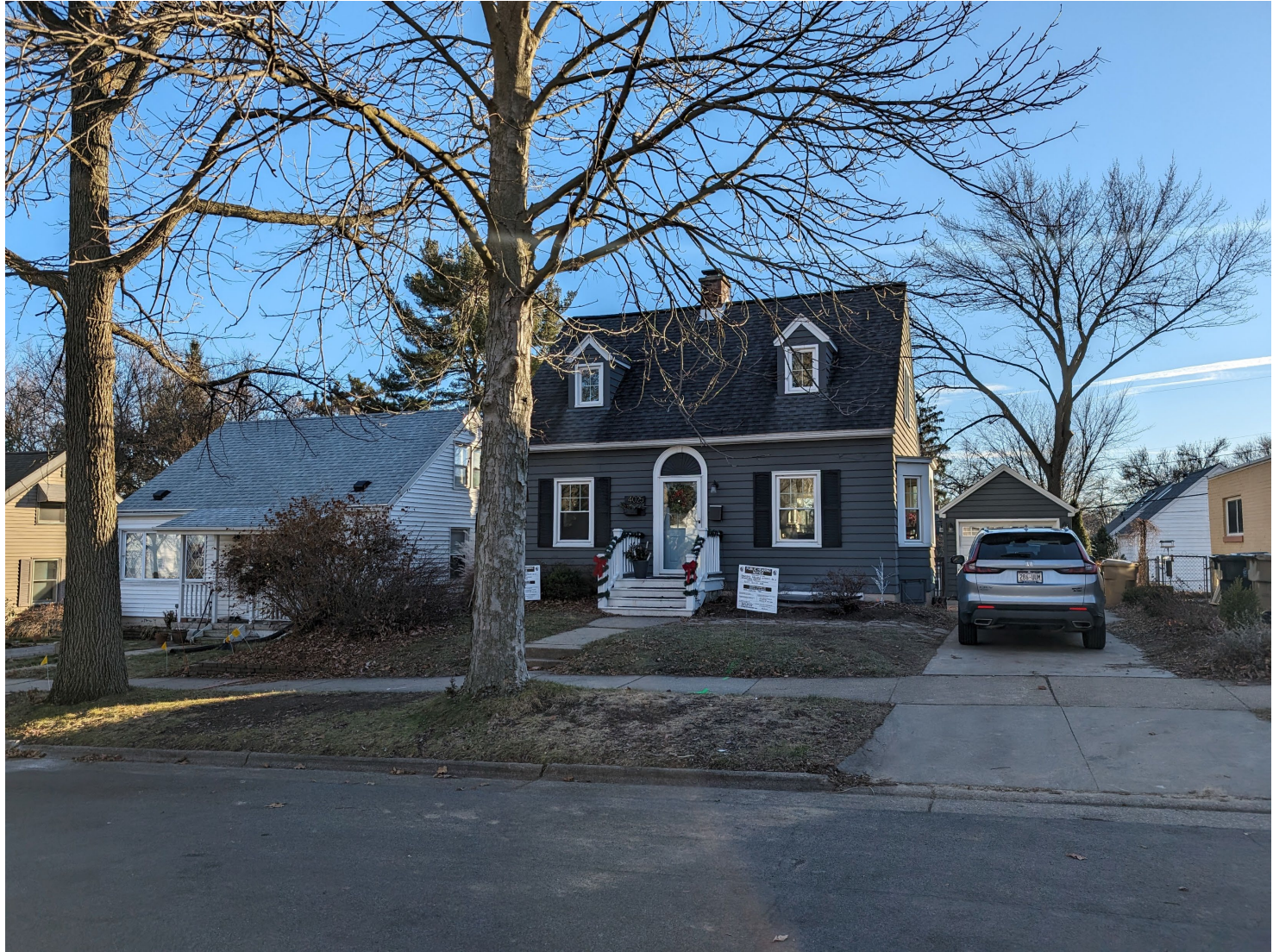
Front North Elevation – View from Birch Ave
