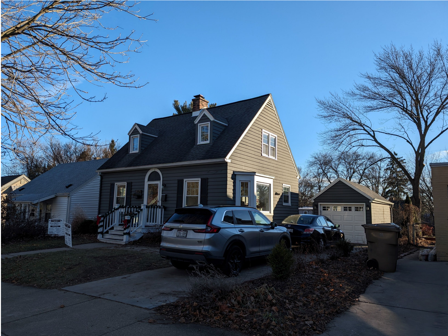
Side West Elevation and Front North Elevation
