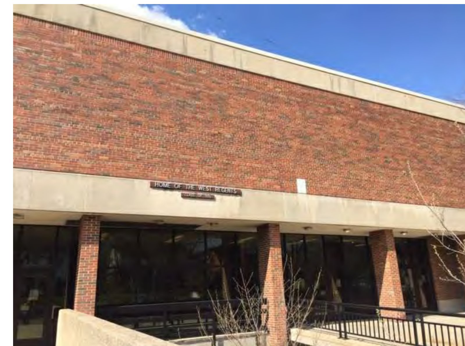
EXISTING BRICK AT GYM
