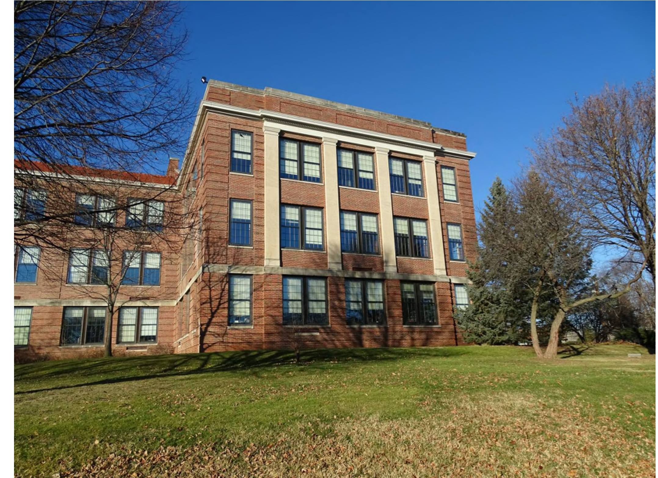
3. VIEW FROM ASH STREET
