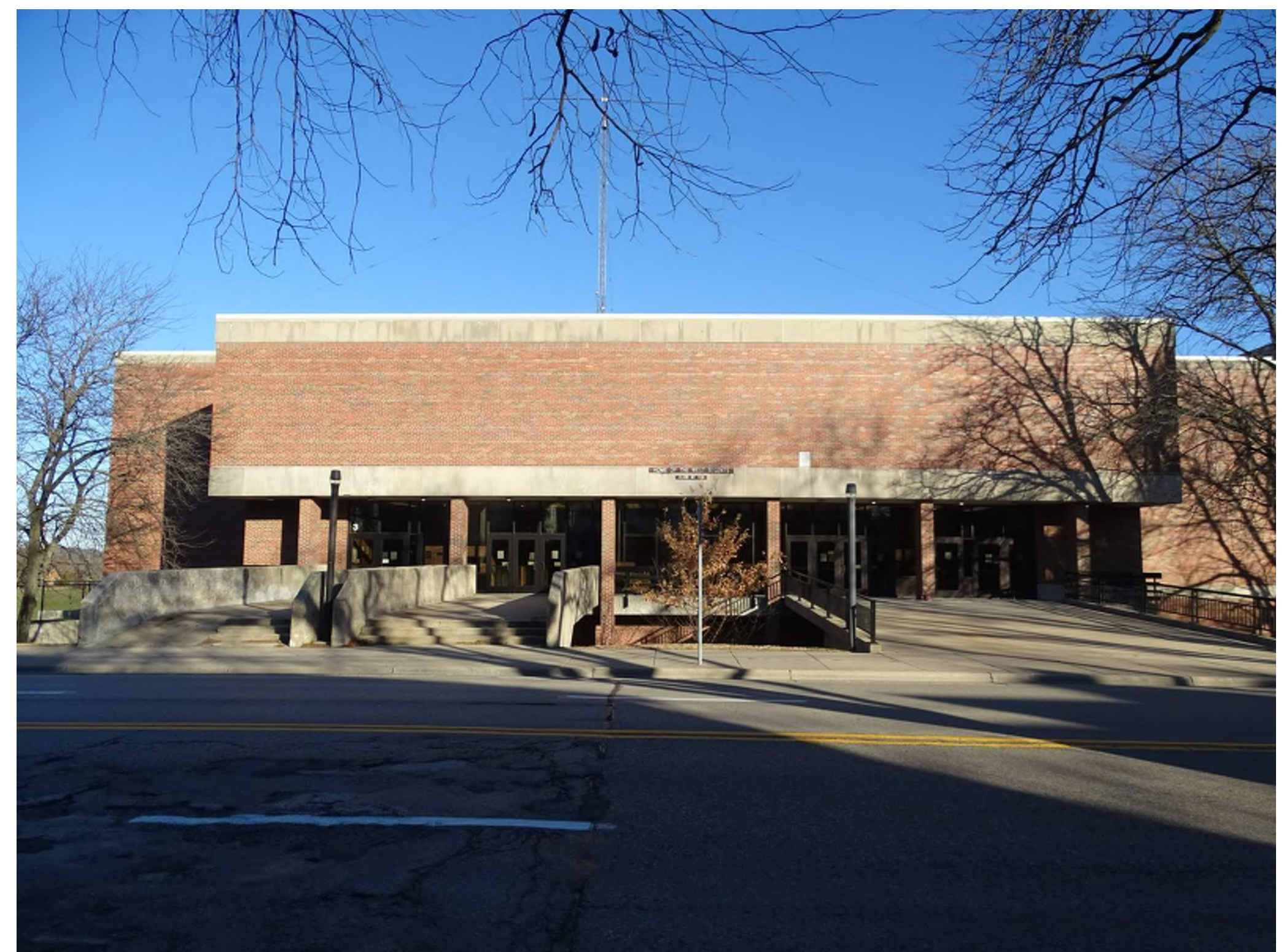
7. VIEW FROM REGENT STREET TO GYM
