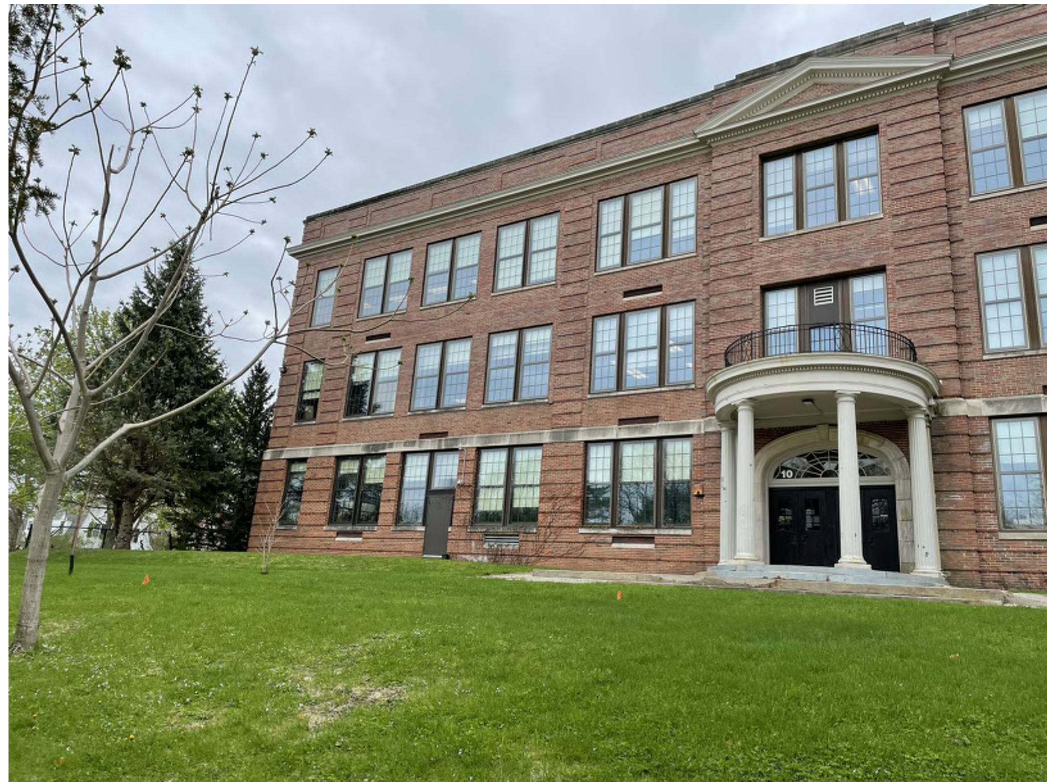
4. VIEW FROM ASH STREET TO NORTH ELEVATION
