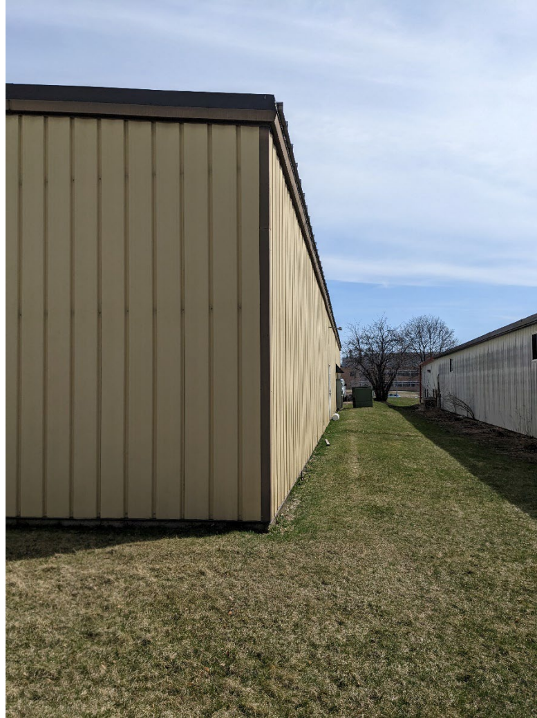
North Side and West Rear Elevation, Looking Towards Pflaum
