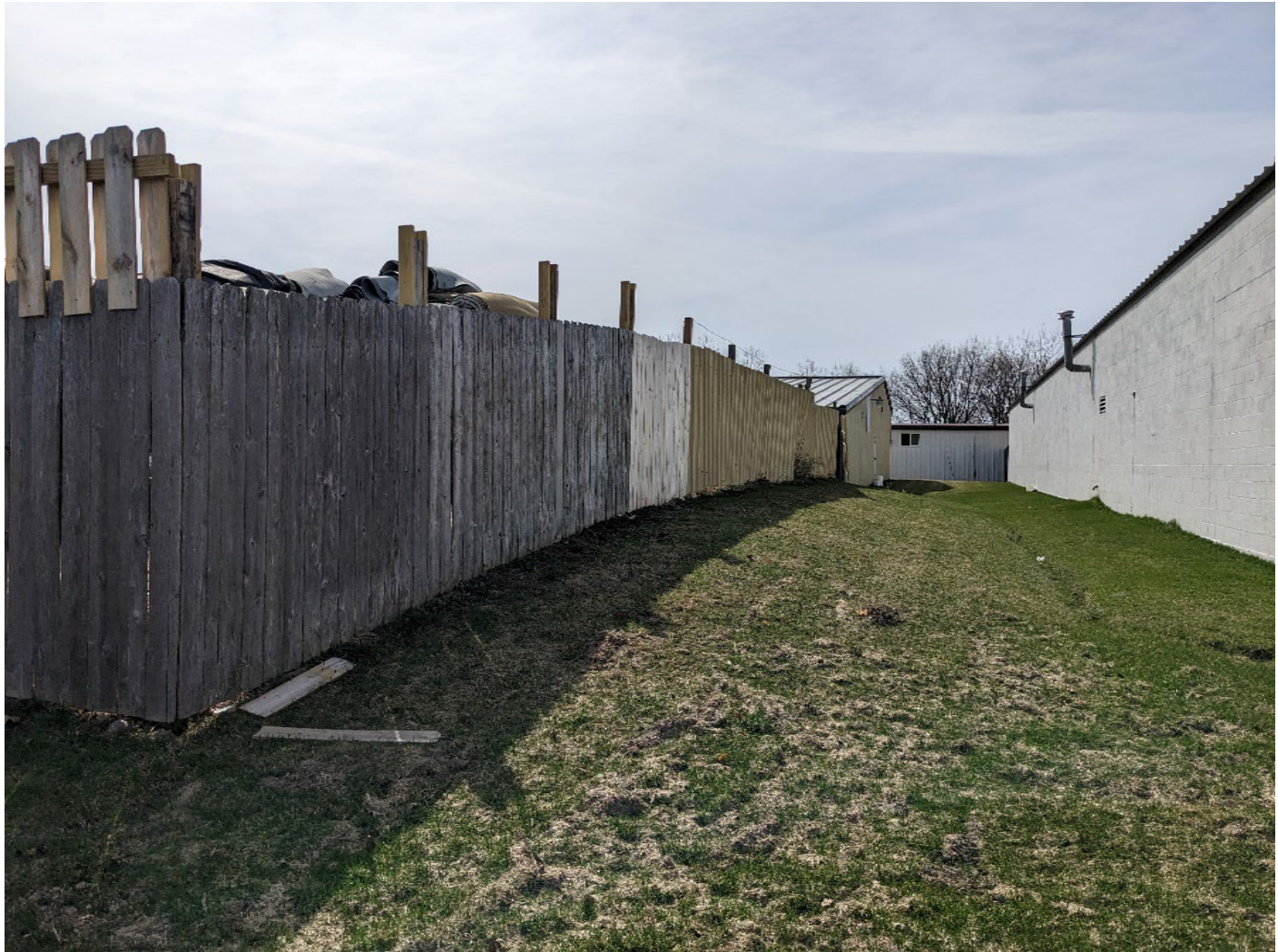
North Side Elevation, Looking Towards Building
