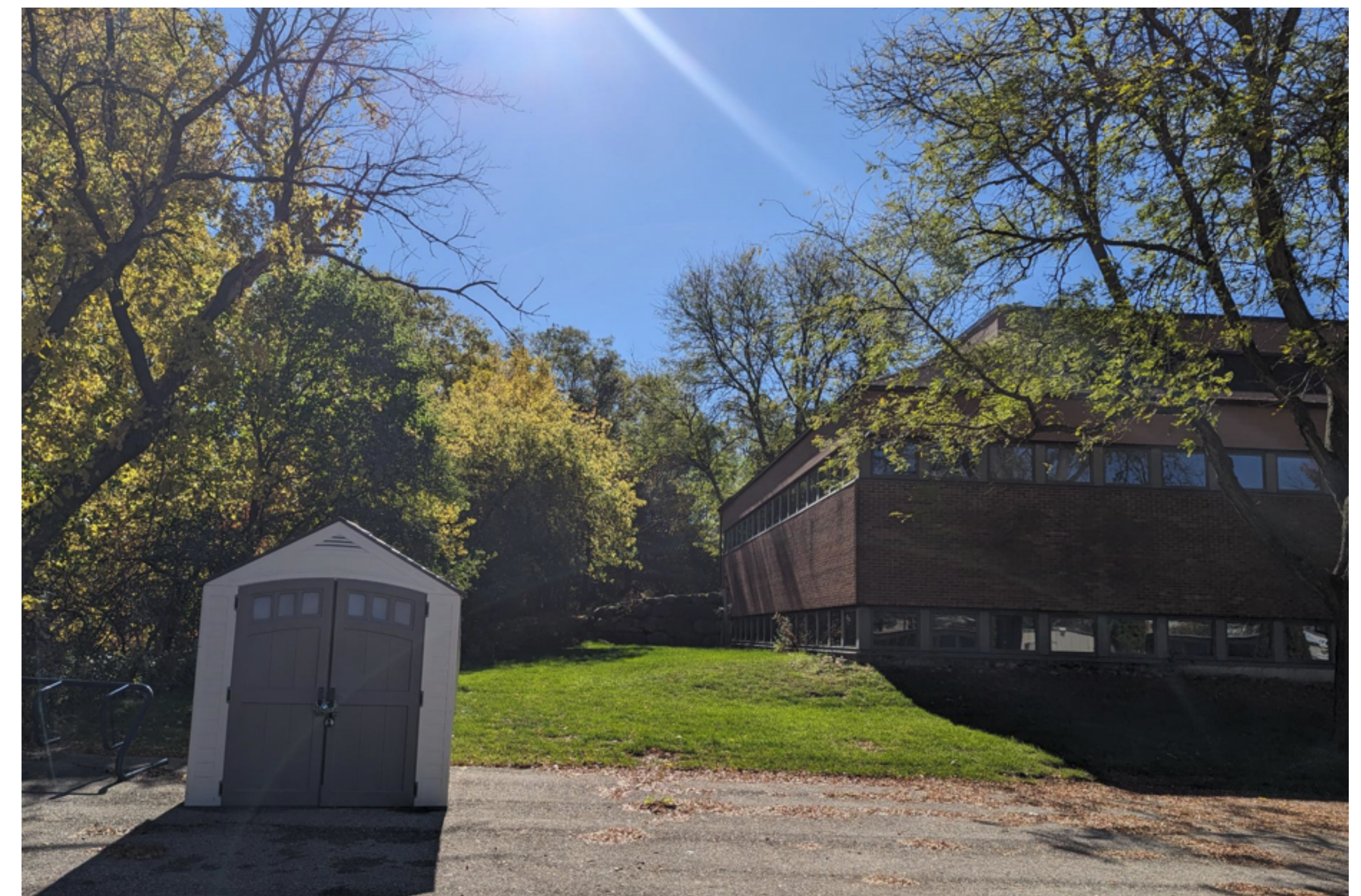
Building to be removed - Exterior photos
