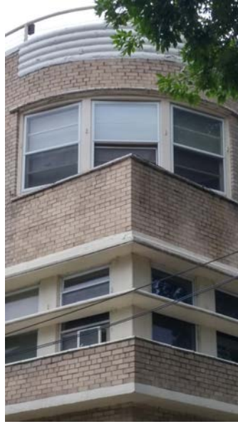
Existing front upper corner windows
