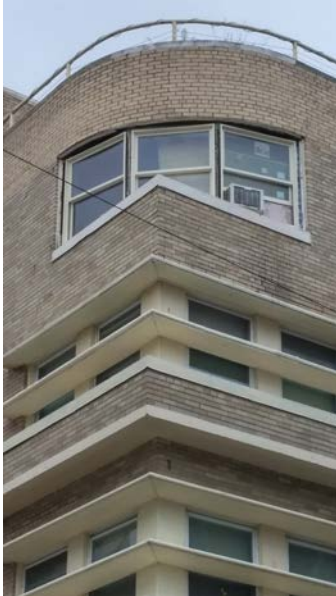
Subject replacement rear upper corner windows
