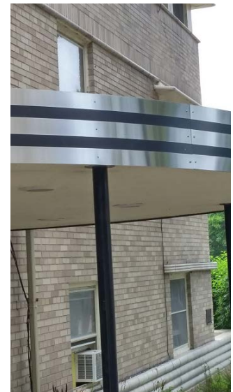
Front entrance canopy fascia
