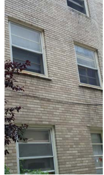
Existing double-hung windows with horizontal muntins
