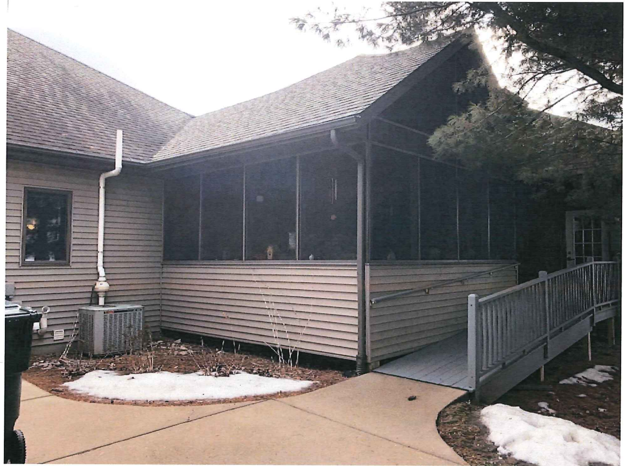
Emerson Senior Living Expansion - Existing Materials
