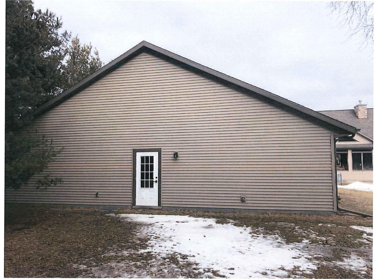
Emerson Senior Living Expansion - Existing Materials
