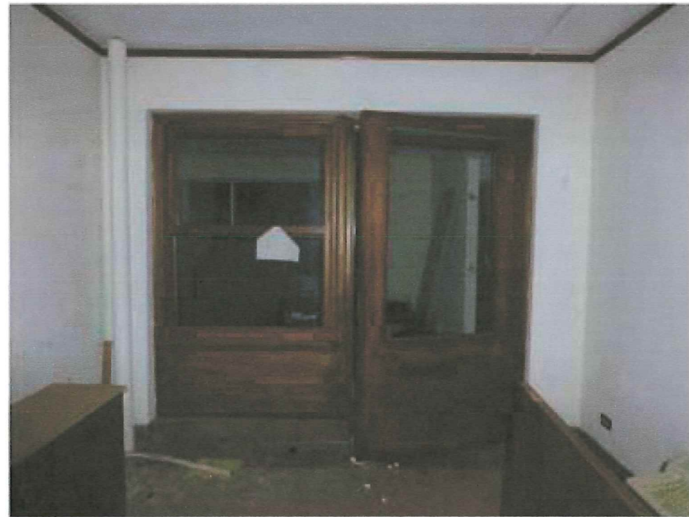
Image 6 Wood door and window, interior, south facing rooms, overall view above
