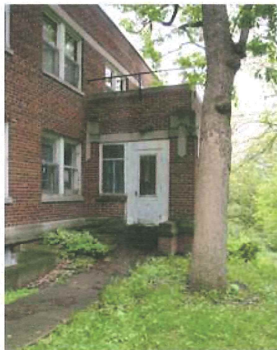
Image 4 Dormitory for Help - Veranda Entrance
