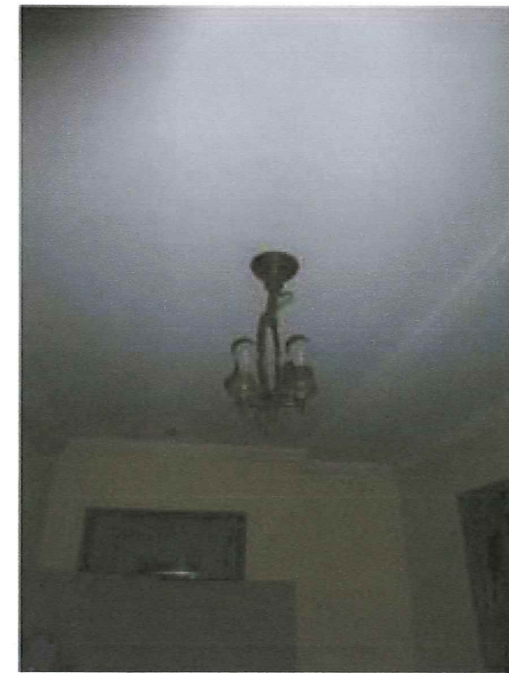
Image 10 Original light fixture, main entry, first floor
