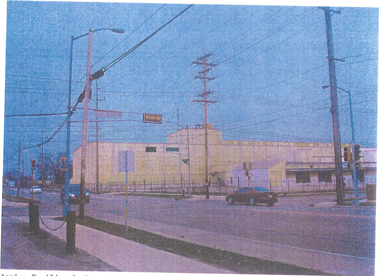
Agrium Facility looking W-NW from Cottage Grove Rd
