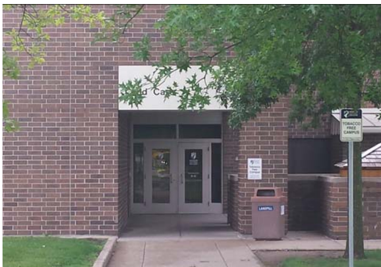
DAY CARE ENTRANCE DOORS
