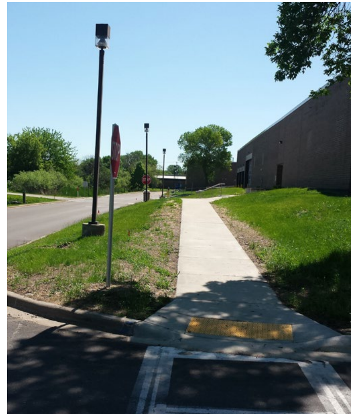
VIEW EAST FROM ENTRY DRIVE
