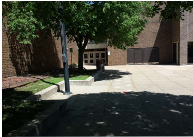
ENTRANCE TO GYMNASIUM STAIRWELL
