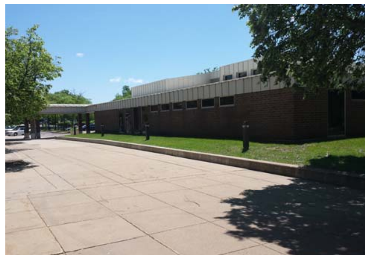
ADMINISTRATIVE BUILDING - NORTH FACE
