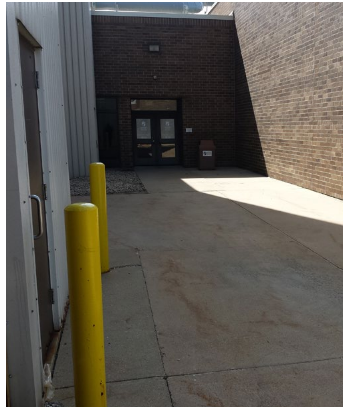
SOUTHWEST CORNER OF LOADING DOCK
