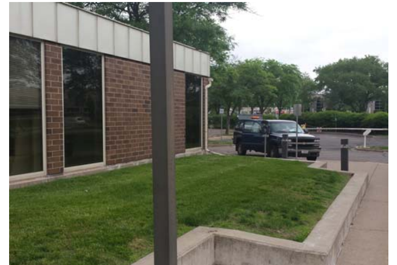
VIEW EAST TO DRIVEWAY EXIT
