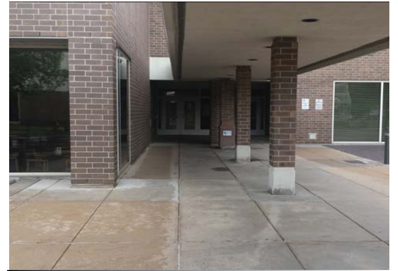
VIEW NORTH TO MAIN ENTRANCE
