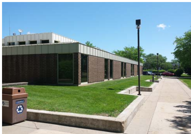
ADMINISTRATIVE BUILDING - SOUTH FACE
