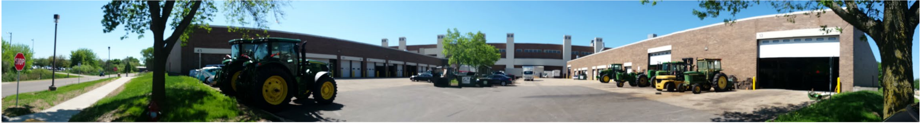
VIEW SOUTH FROM ENTRY DRIVE
