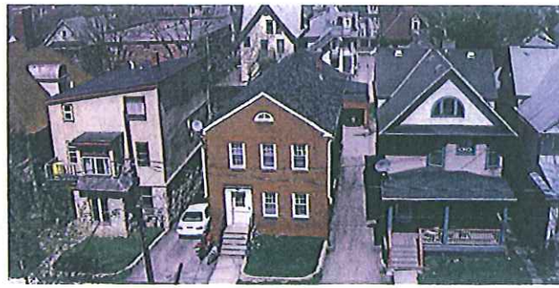
The three existing buildings at 119, 123 & 125 N, Butler. The building on right will be moved to 520 East Johnson and the two buildings to the left will be demolished
