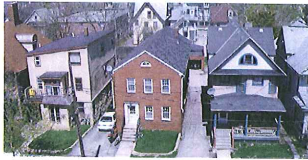
The three existing buildings at 119, 123 & 125 N. Butler. The building on right will be moved to E. Johnson and the two buildings on the left will be demolished
