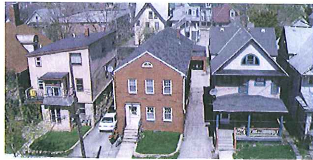
The three existing buildings at 119, 123 & 125 N, Butler. The building on the right will be moved to E. Johnson and the two buildings on the left will be demolished
