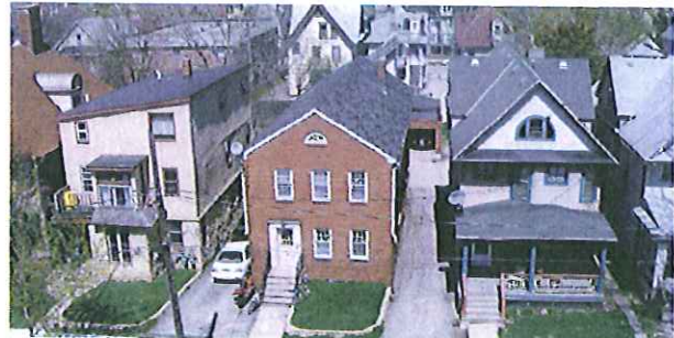
The three existing buildings at 119, 123 & 125 N, Butler. The building on the right will be moved to E. Johnson and the two buildings on the left will be demolished
