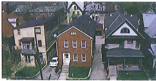
The three existing buildings at 119, 123 & 125 N, Butler. The building on right will be moved to 520 East Johnson and the two buildings to the left will be demolished
