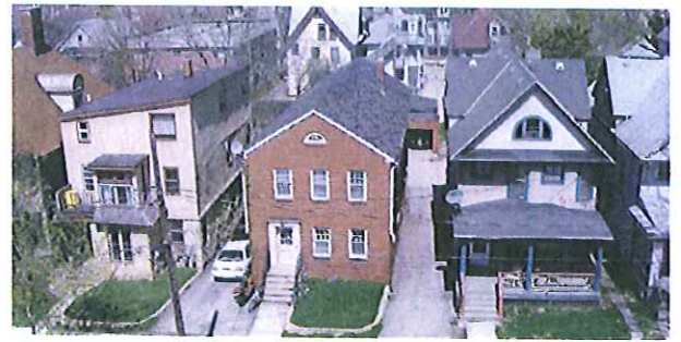
The three existing buildings at 119, 123 & 125 N, Butler. The building on right will be moved to E. Johnson and the two buildings on the left will be demolished
