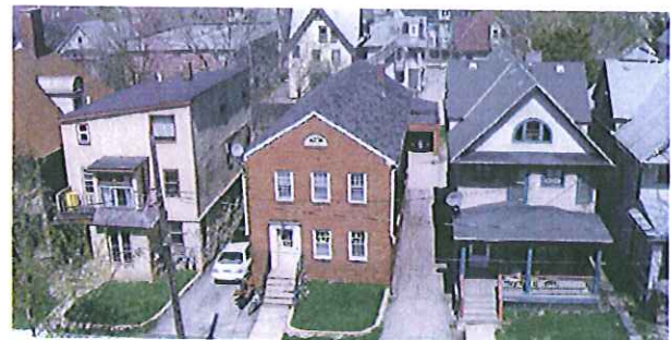
The three existing buildings at 119, 123 & 125 N. Butler. The building on the right will be moved to E. Johnson and the two buildings on the left will be demolished
