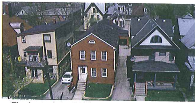
The three existing buildings at 119, 123 & 125 N. Butler. The building on right will be moved to 520 East Johnson and the two buildings to the left will be demolished
