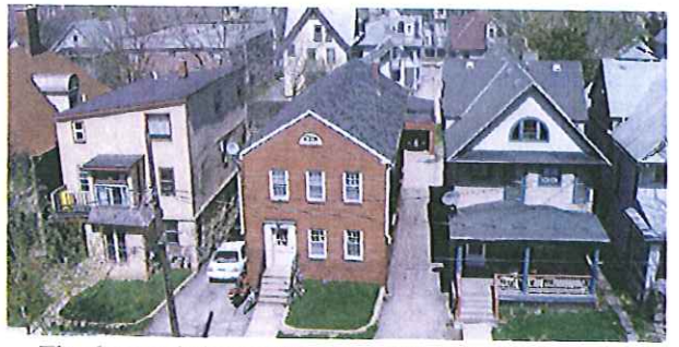
The three existing buildings at 119, 123 & 125 N. Butler. The building on right will be moved to E. Johnson and the two buildings on the left will be demolished
