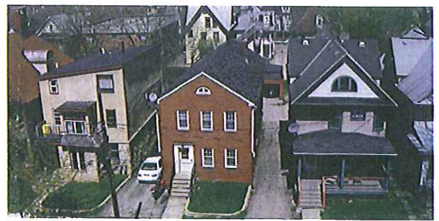
The three existing buildings at 119, 123 & 125 N, Butler. The building on right will be moved to 520 East Johnson and the two buildings to the left will be demolished
