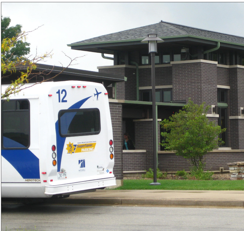
The train station located at General Mitchell International Airport in Milwaukee is fully ADA compliant, with all resources and amenities meeting current standards.
