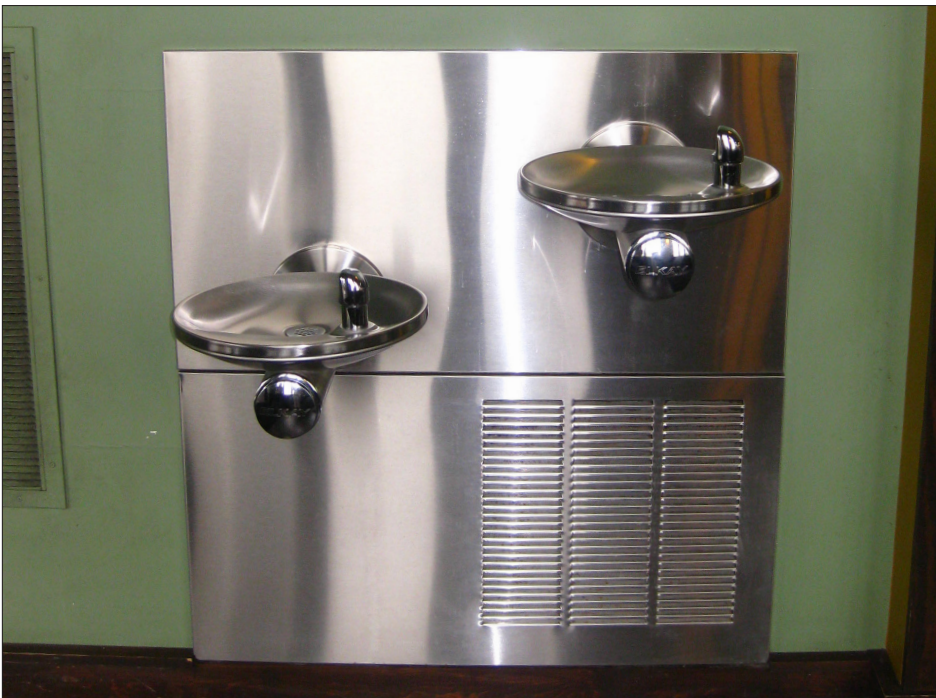
ADA-compliant “hi-lo” drinking fountains include one fountain that is accessible to those who use wheelchairs and one fountain installed at a standard height that is convenient for those who have difficulty bending.
