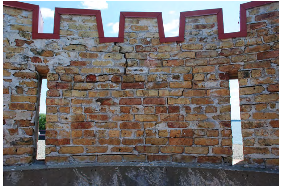
Existing Conditions Machinery Row Turret Replacement July 15, 2014
