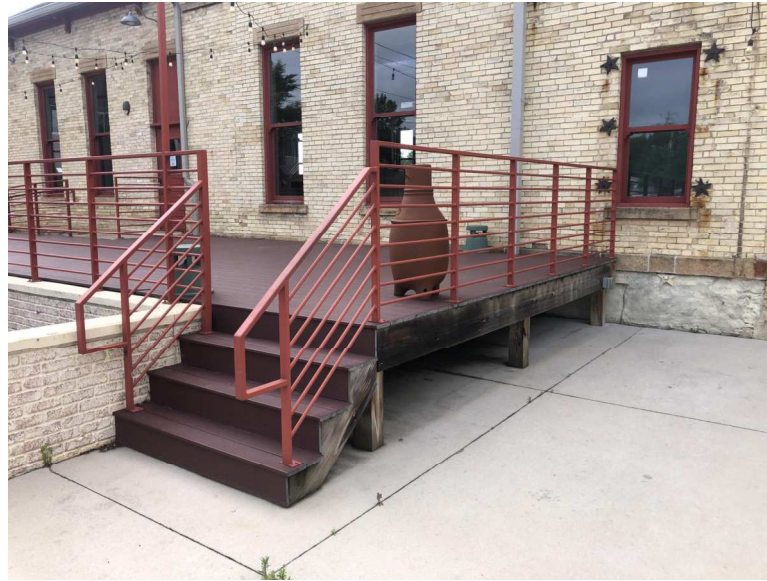
Existing Patio and Porch
