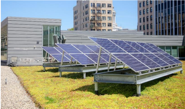
Solar Installations & Green Roofs
