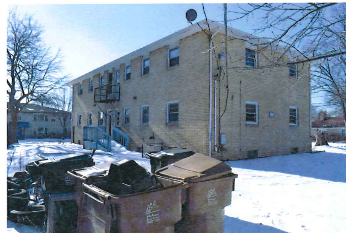
EAST ELEVATION, LOOKING SOUTHWEST
