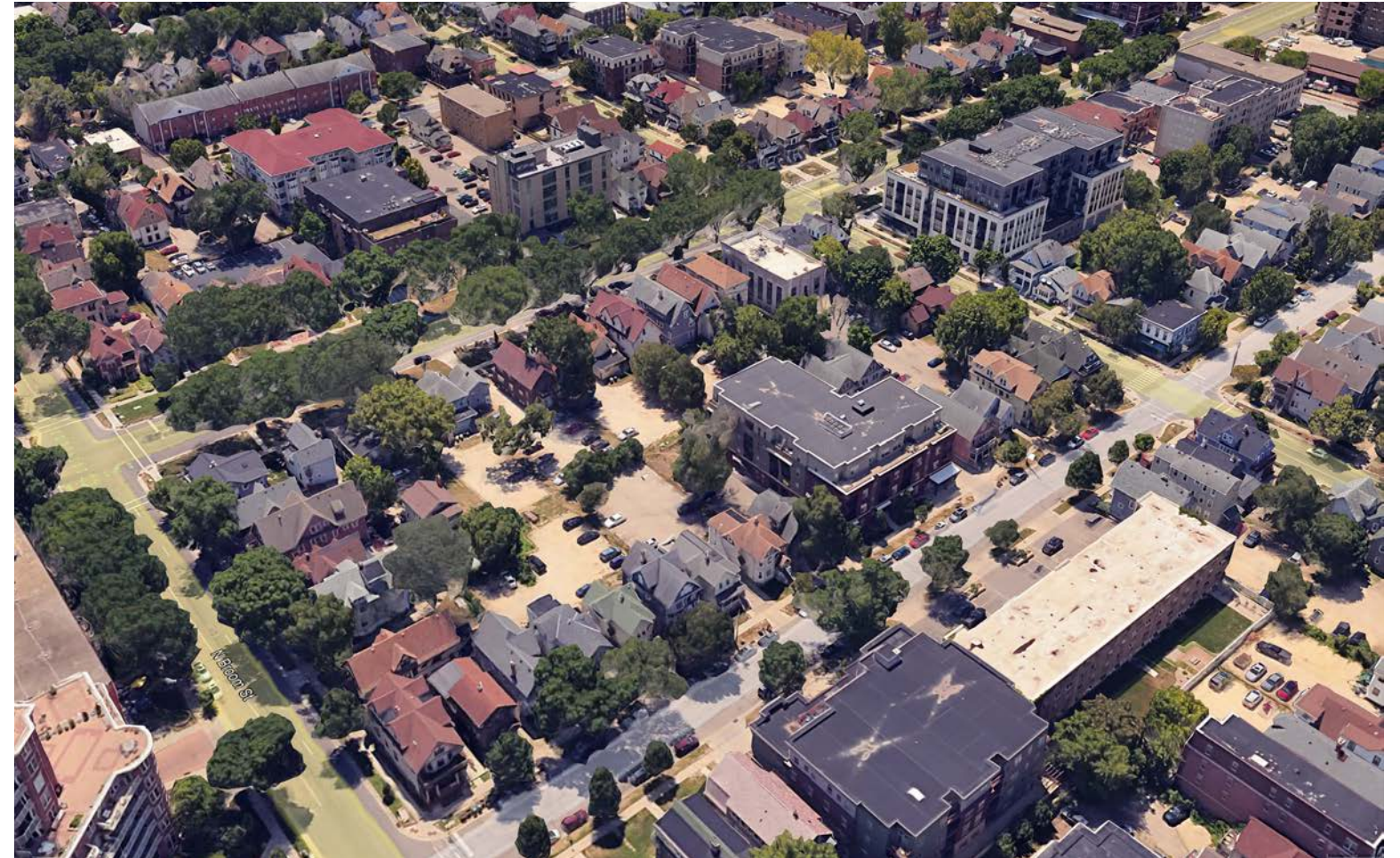
Aerial View - Mifflin St.
