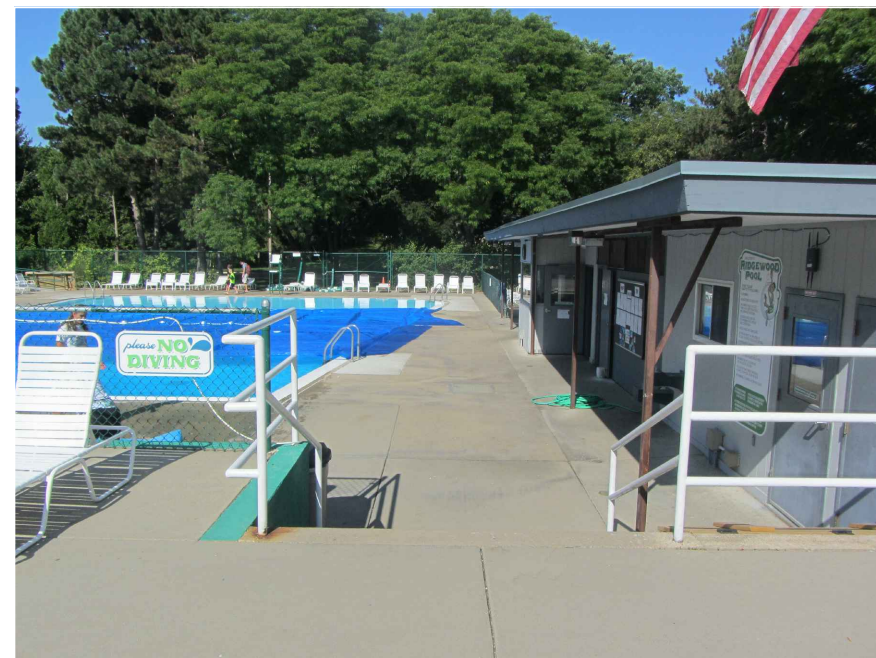
POOL DECK AND POOL HOUSE FROM EAST
