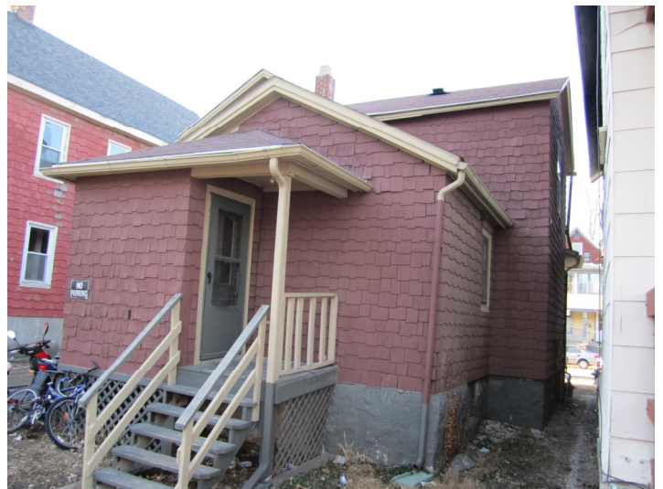
531 Mifflin existing building— from southeast
