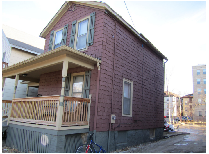
531 Mifflin existing building— from west
