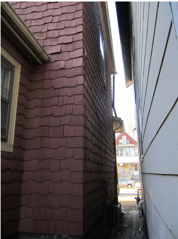
531 Mifflin existing building— northeast condition
