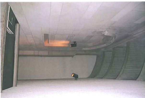
9. SKYLIGHTS OVER SW CORNER OF CHAPEL
