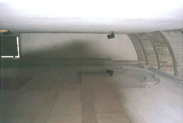
8. SKYLIGHTS OVER SE EXIT OUT OF CHAPEL
