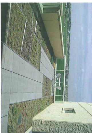
24" x 24" CONCRETE PAVERS ARE USED ON THE GREEN ROOF TO PROVIDE SAFE PEDESTRIAN ACCESS. THE PAVERS ARE SPACED 1/4" FROM THE ADJACENT PLANTS. COLOR FOR THE 24" SQUARE PAVERS WILL COMPLEMENT THE BUILDING.
