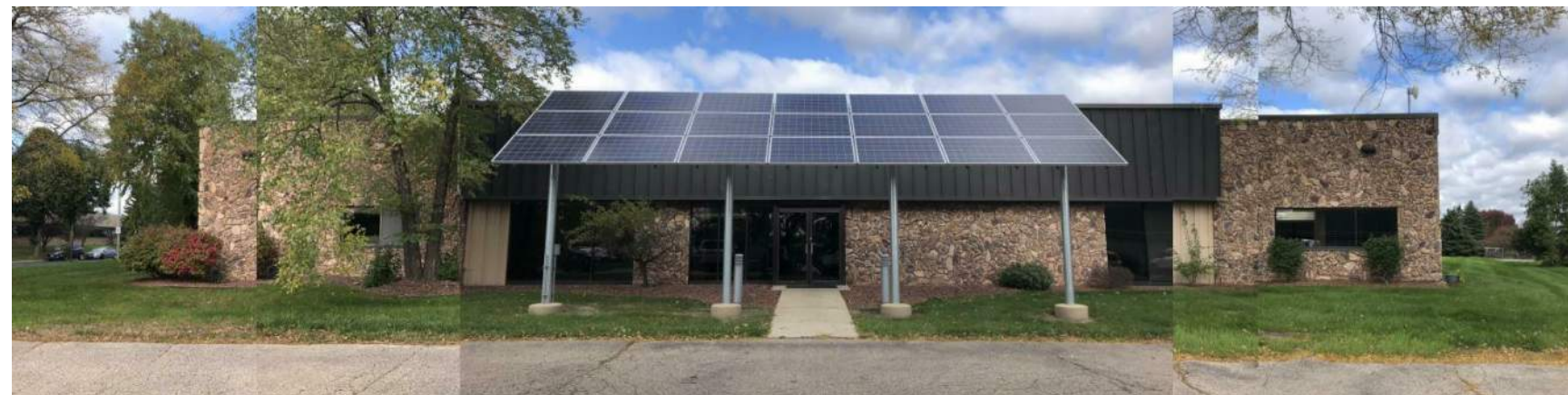
SOUTH ELEVATION - EXISTING PHOTOS
