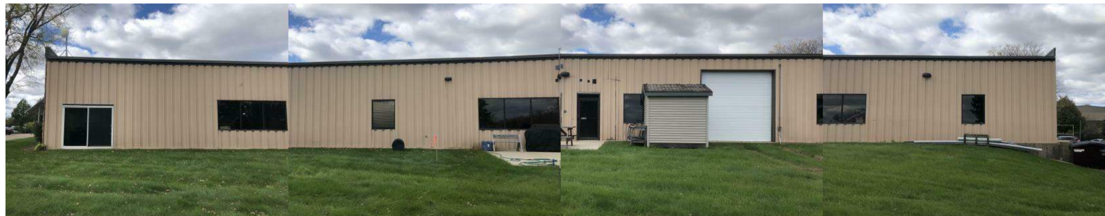
EAST ELEVATION - EXISTING PHOTOS
