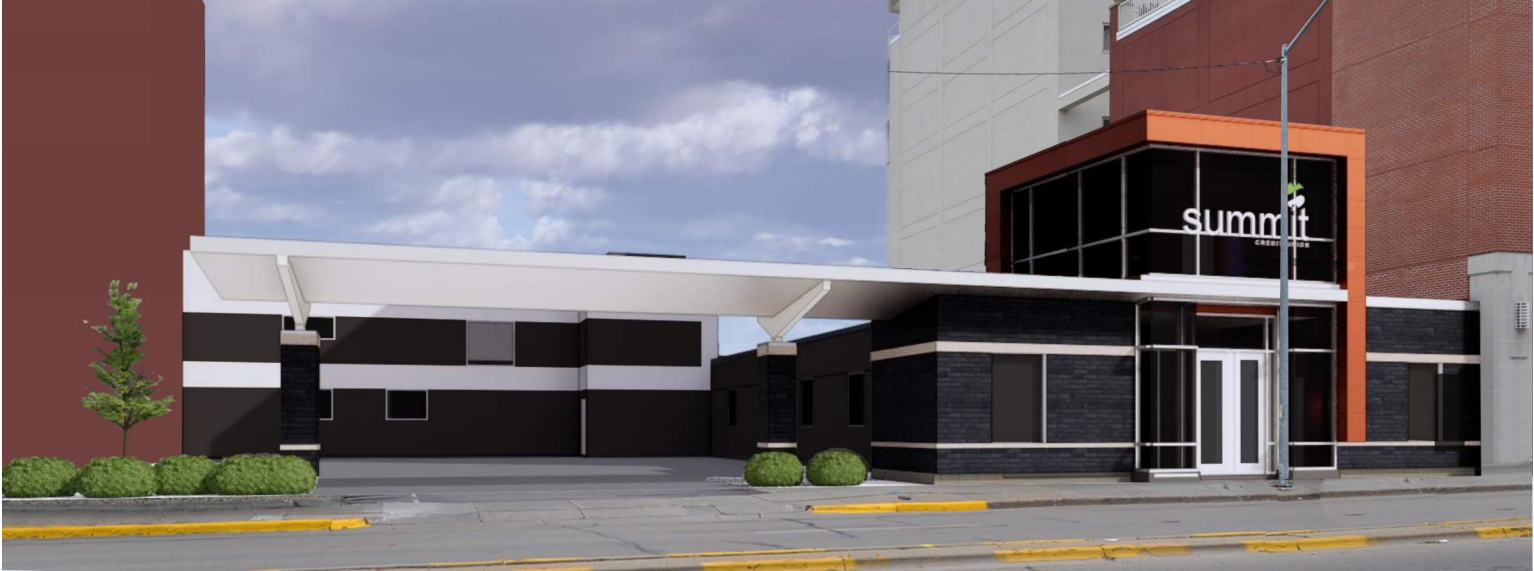
WILSON ST. FACADE
