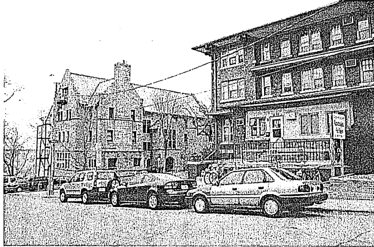
625-31 N. Henry (building on right) – proposed for demolition & 150 lota Court
