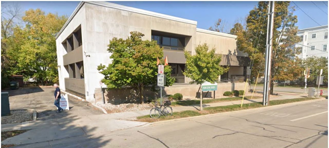
8) View looking Southeast from W Wilson St
