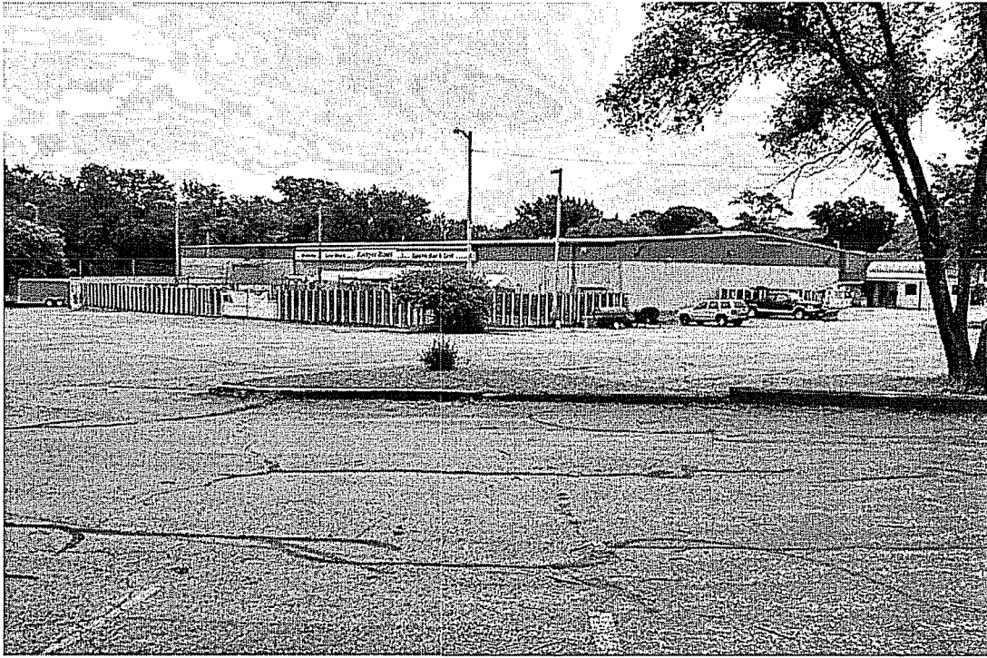
Northwest portion of site and building
