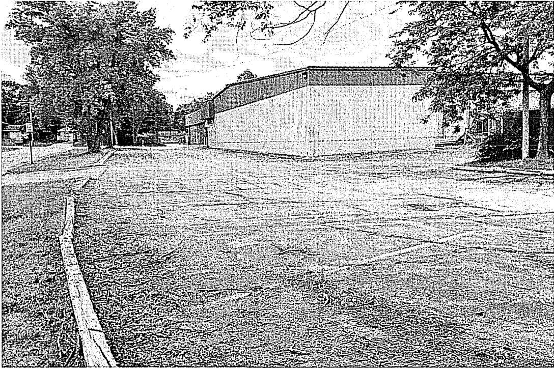
East Elevation. Rear of building
