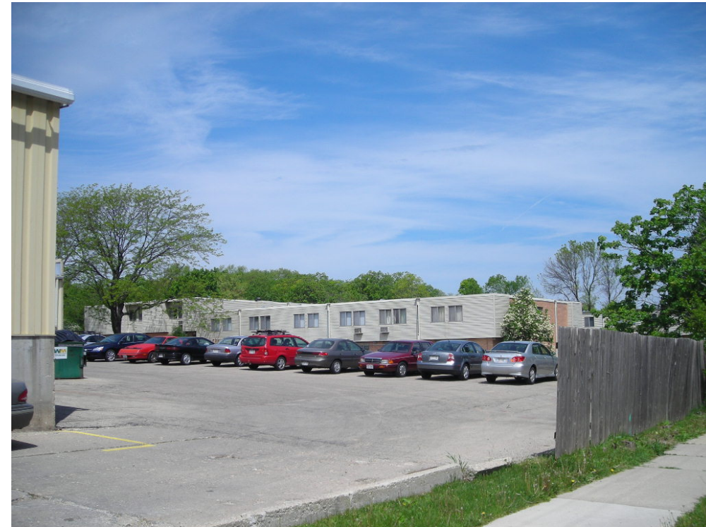
View North at Existing Apartments
