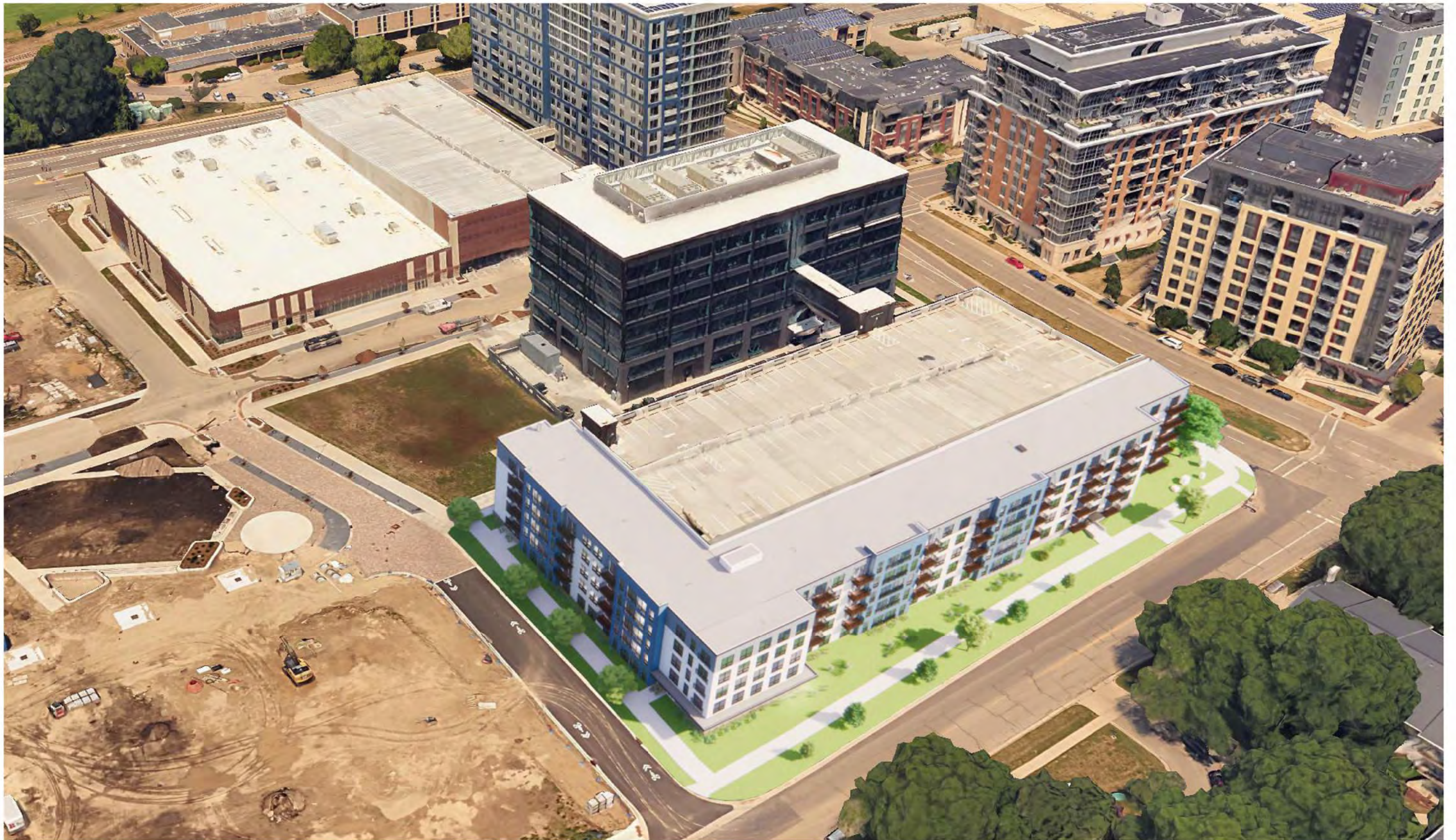
AERIAL VIEW FROM SHEBOYGAN AVENUE LOOKING NORTHEAST
