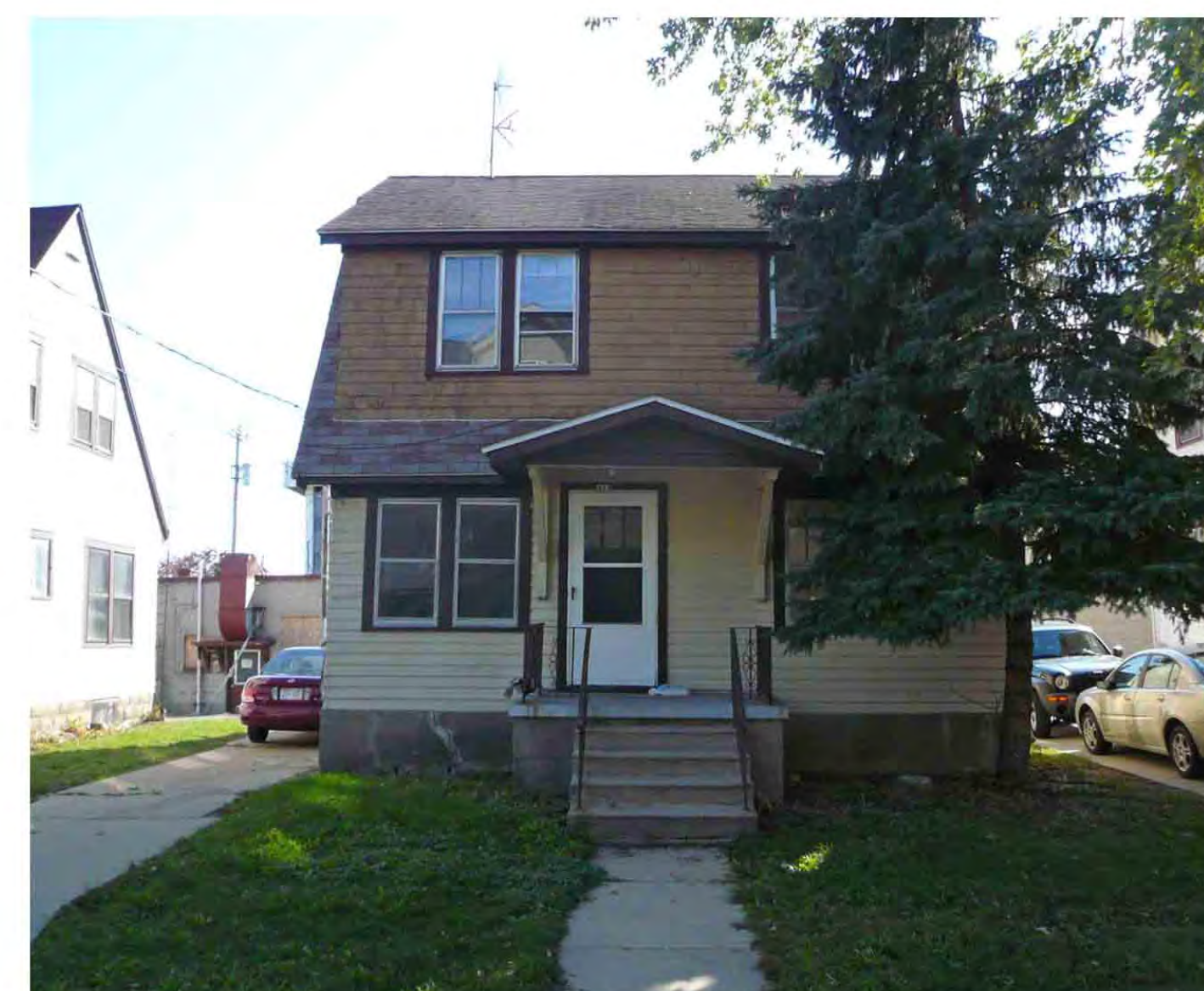
College Court: Looking South
