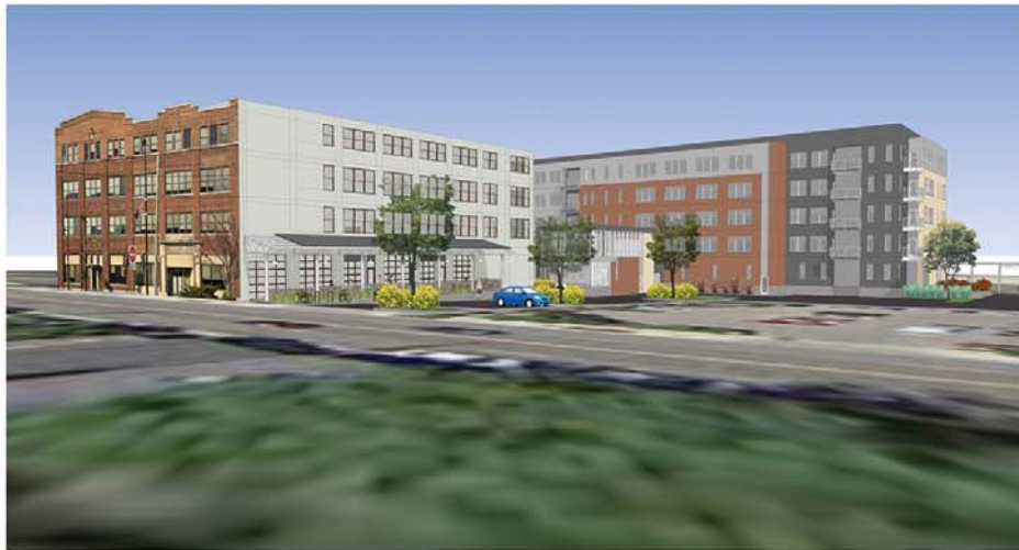
View from Williamson Street
