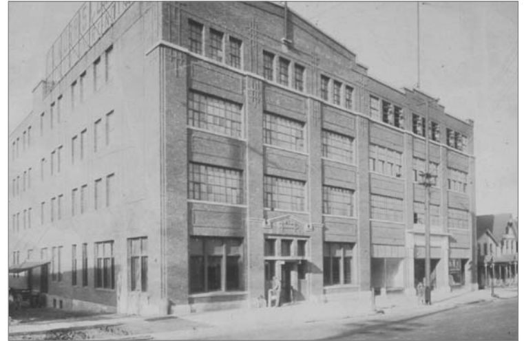
Early Photos of Williamson Street Elevation
