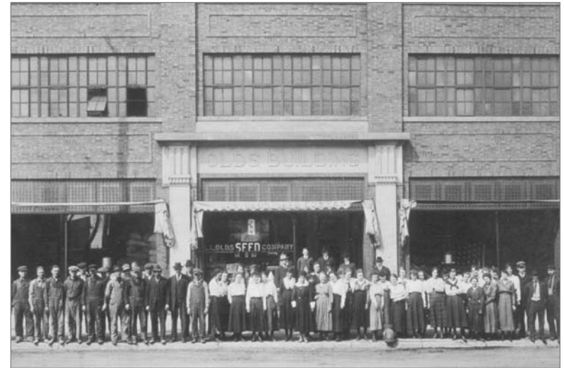
Early Photos of Williamson Street Elevation
