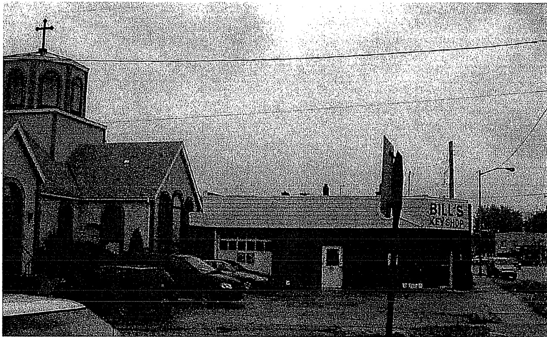
Photo 6: Overall view of Assumption Greek Orthodox Church relative to former Bill's Key Shop, looking east along East Washington Ave. Demolition of building will allow full view of Church from East Washington Ave, increased greenspace, and restoration of parking stalls in accordance with the City.
