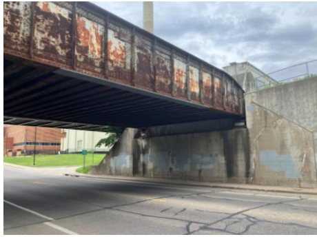
The railroad bridge beyond the project boundary
