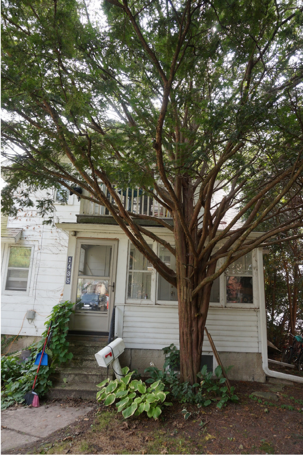
Exterior of house - Street side of house close shot
