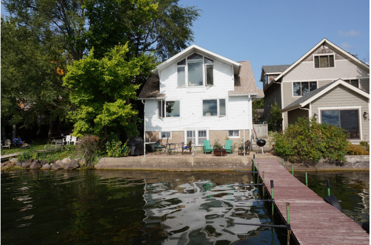
Exterior of House - Lake side of house
