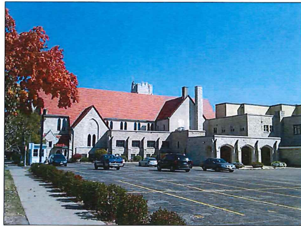
4 A100 VIEW TO INTENDED SITE
