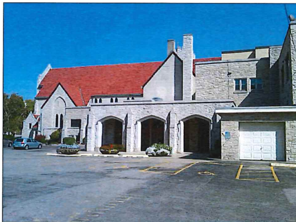
3 A100 VIEW TO INTENDED SITE
