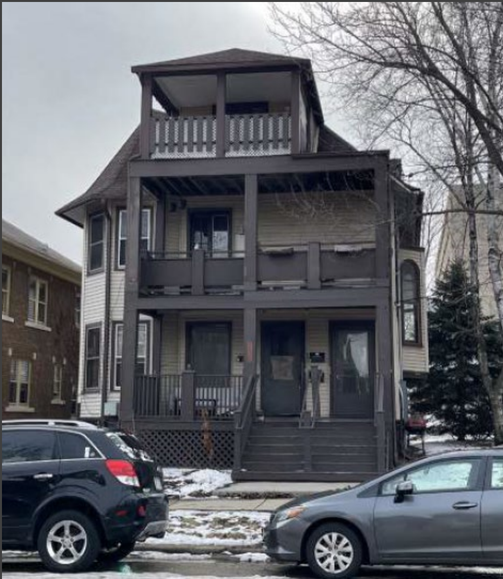
Existing Hancock Street or North Elevation
