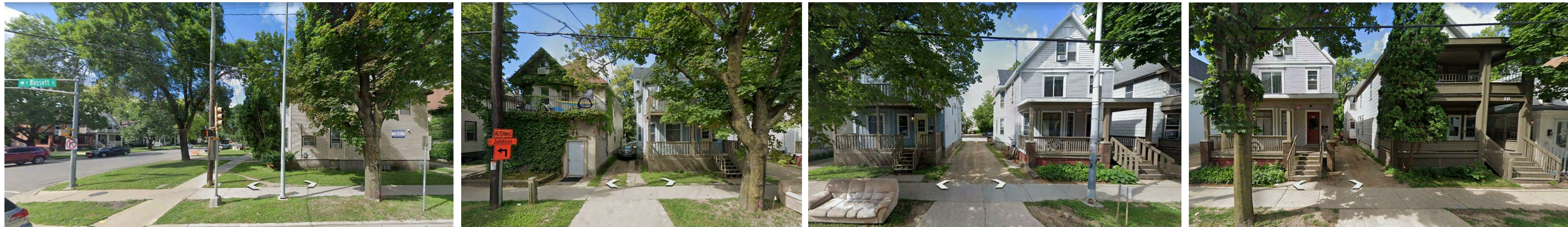
NORTH BASSETT STREET EXISTING CONDITIONS
