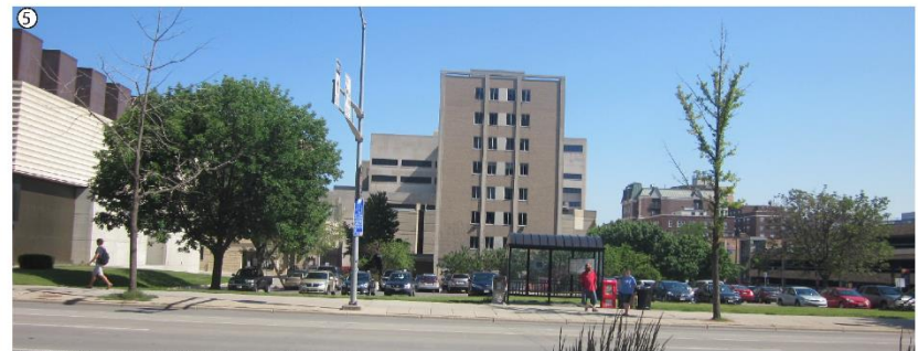
Panoramic View Northeast from the Lucky Apartments
