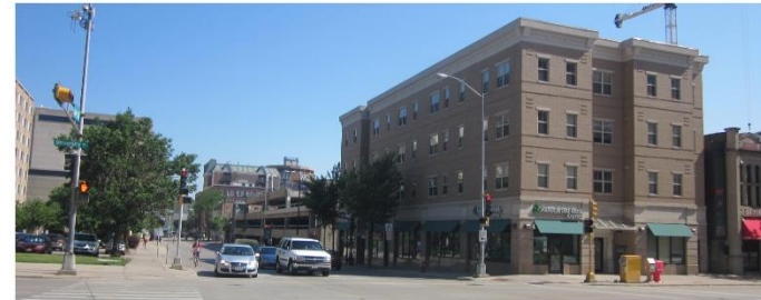
Site Approach Corner Associated Bank Building
