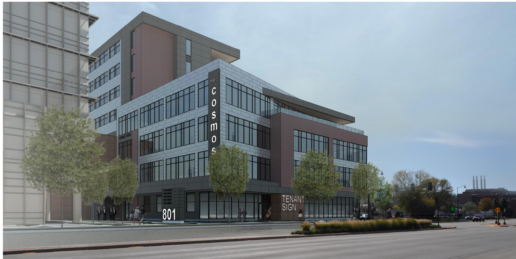
VIEW FROM E. WASHINGTON (LOOKING SW) - TOWER ALTERNATE
