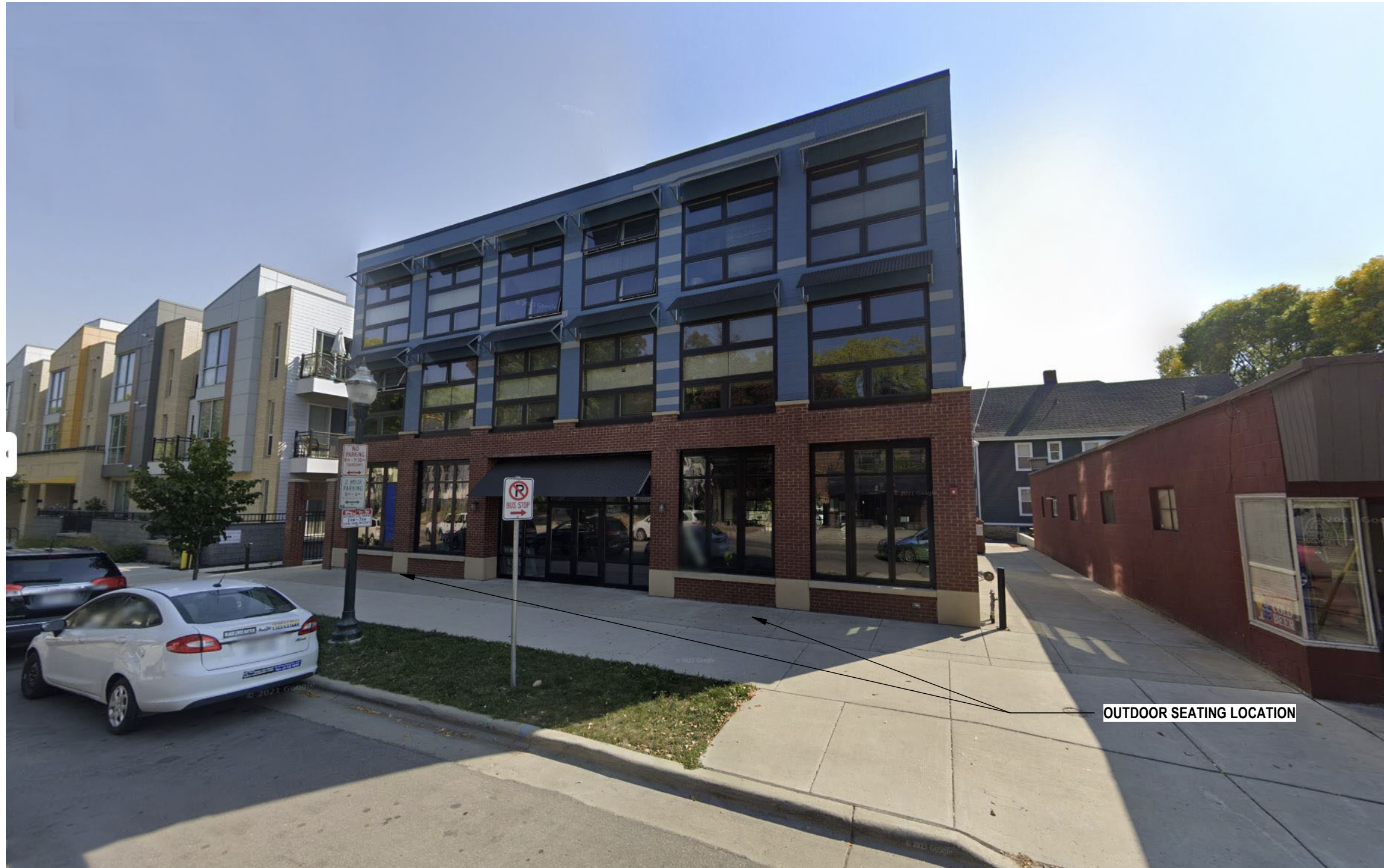
EXISTING EAST JOHNSON BUILDING FACADE
