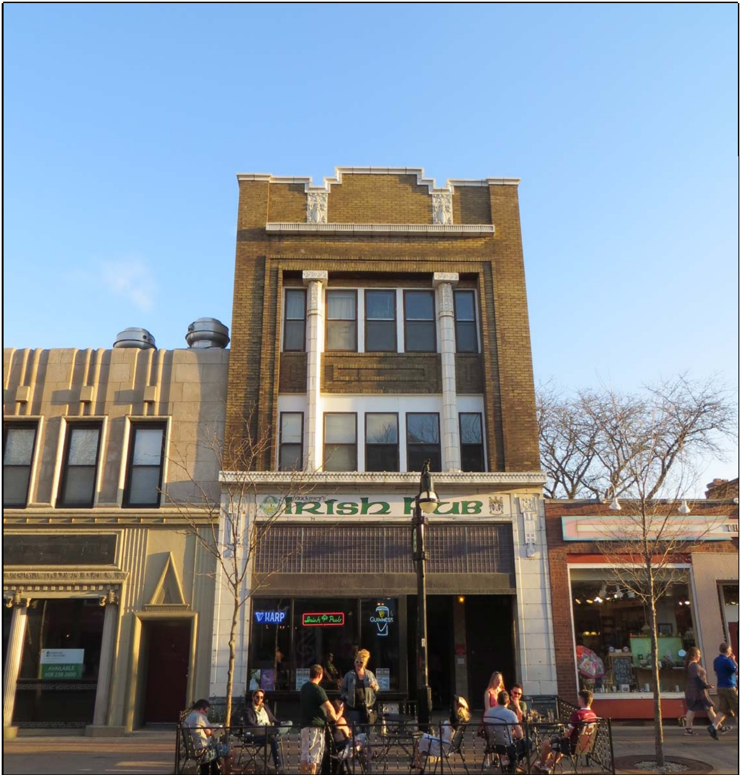
Photo 1 - VIEW OF PRIMARY FAÇADE FROM STATE ST (NO ANTENNA VISIBILITY)
