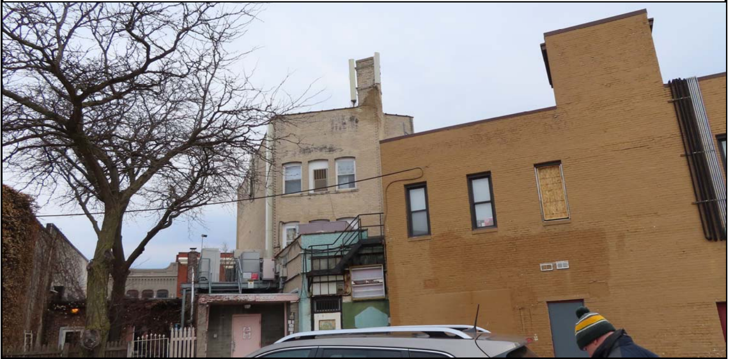
Photo 8 - ALTERNATE VIEW OF ANTENNAS ON CHIMNEY FROM BEHIND BUILDING
