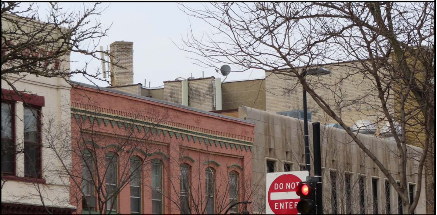
Photo 11 - ZOOMED DETAIL VIEW OF ANENNAS ON EAST WALL OF BUILDING FROM SAME LOCATION AS PREVIOUS
