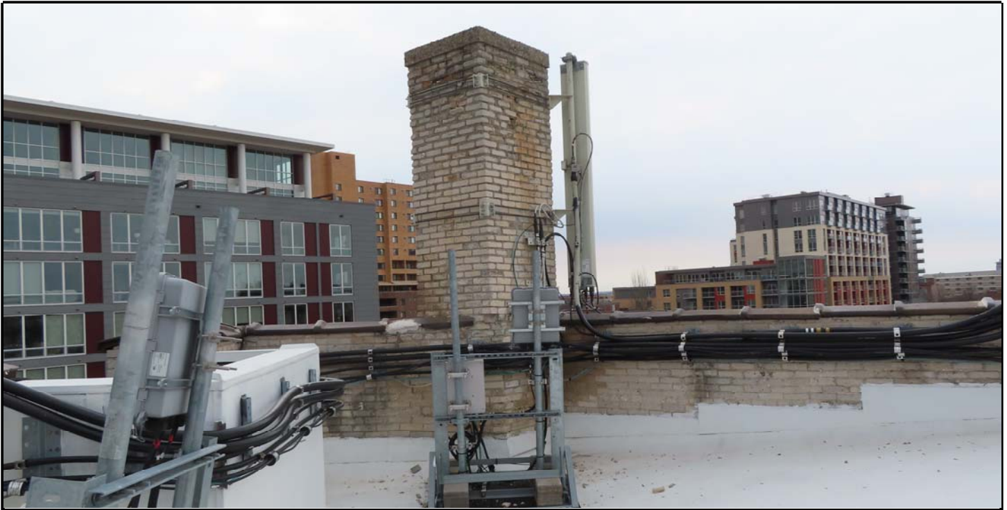
Photo 7 - EXISTING ANTENNAS ON CHIMNEY AT SOUTH SIDE OF ROOF (FROM ROOF)
