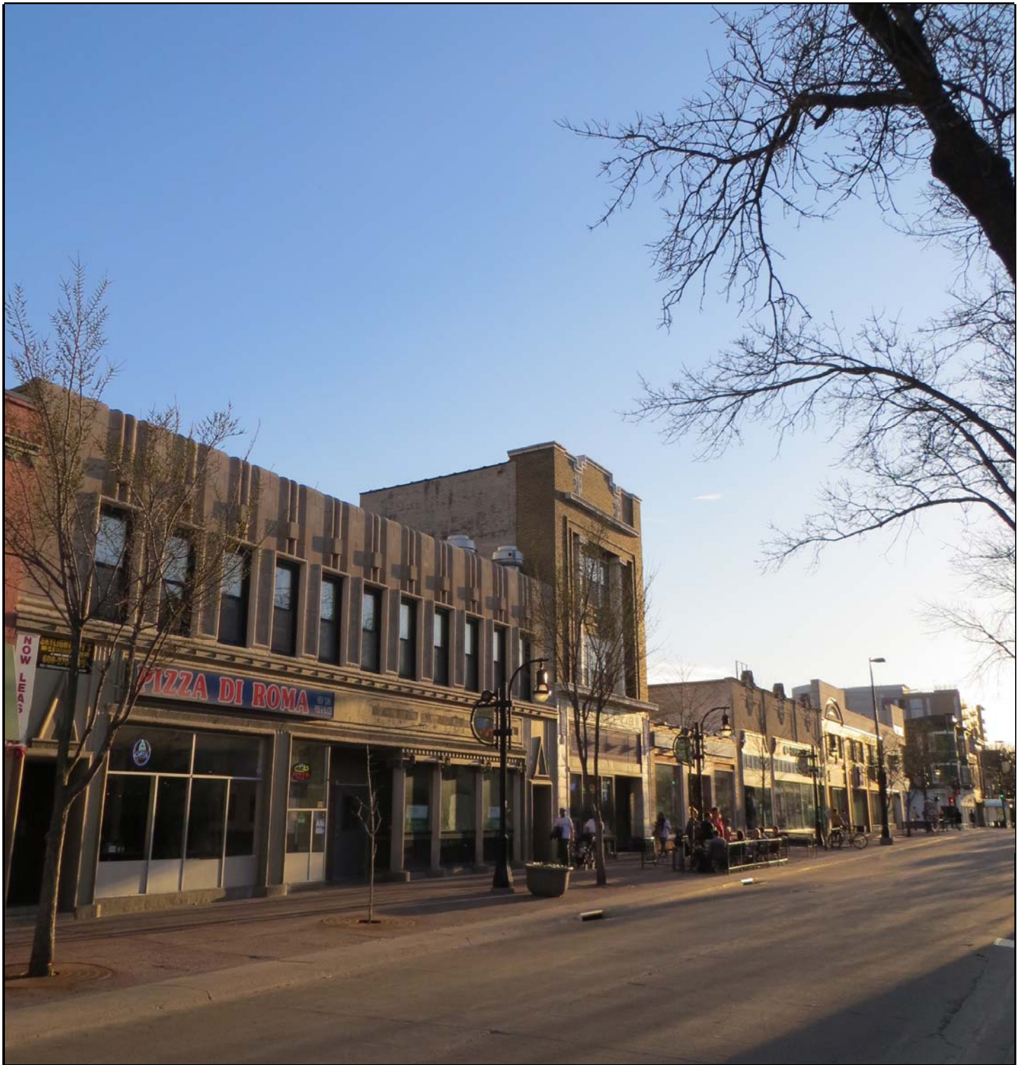
Photo 9 - VIEW OF PRIMARY STRUCTURE FROM STATE ST (NO ANTENNA VISIBILITY)
