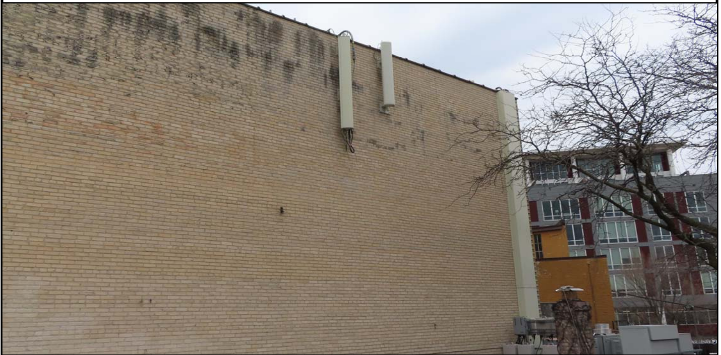
Photo 3 - EXISTING ANTENNAS ON WEST WALL (CAN BE VISIBLE FROM STREET IN SOME AREAS)
