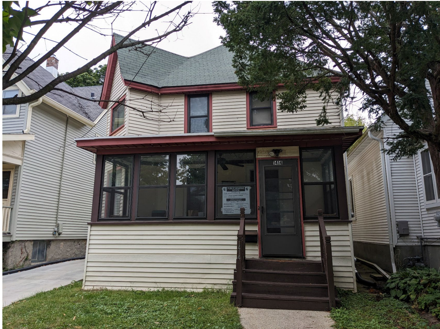
South Front Elevation – View from Jenifer St
