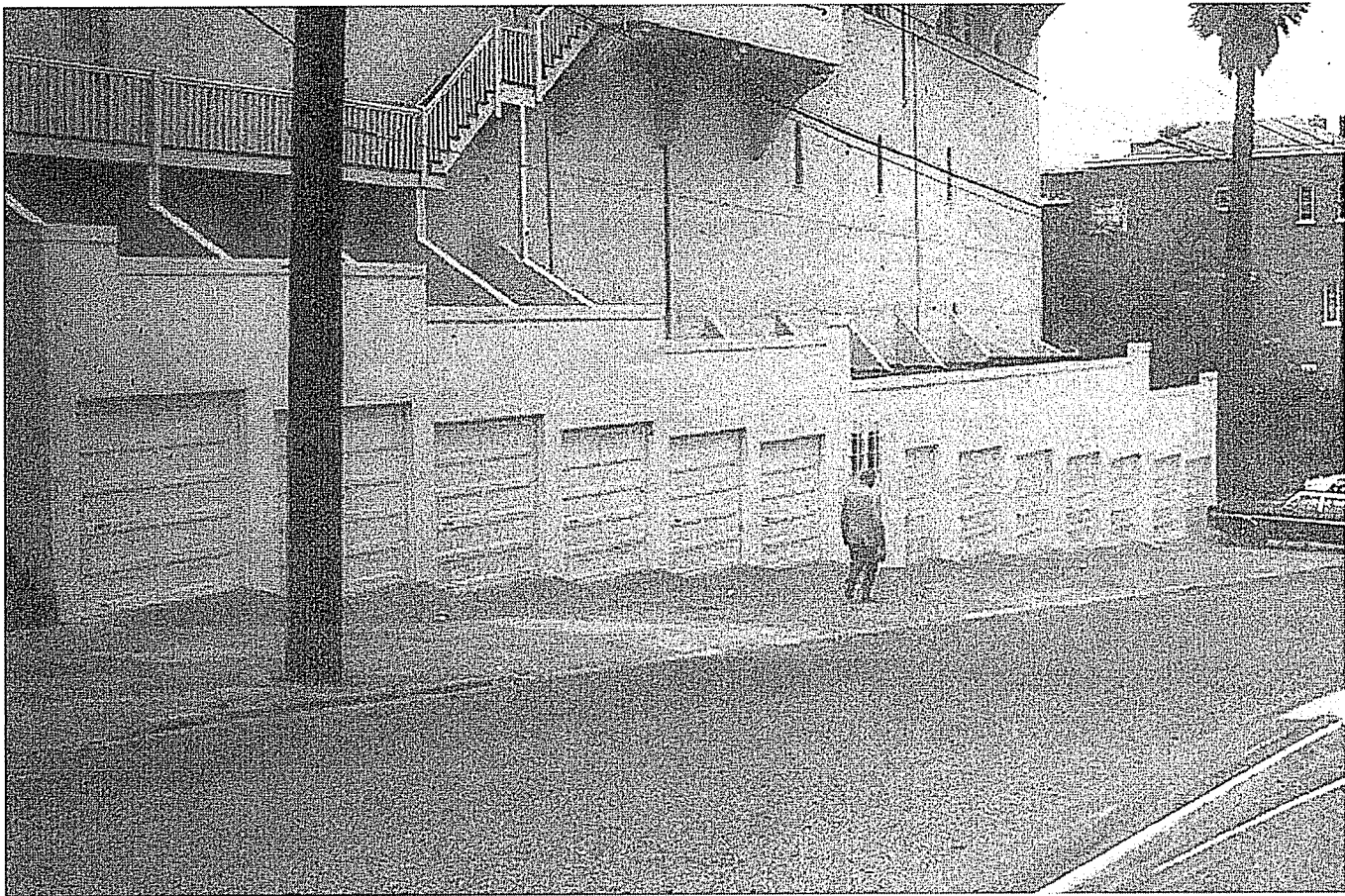
Figure 2. Off-street parking in San Francisco. Source: San Francisco Planning Department
