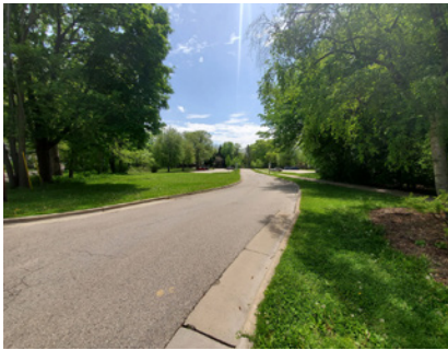
Figure 5.40. North Entry to Parking Lot
