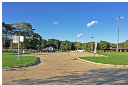
Figure 5.44. Main Shelter Parking Lot
