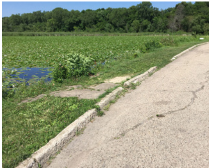
Figure 5.32. Drain Trench to Lake
