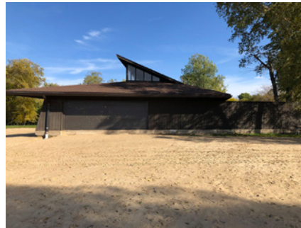
Figure 5.9. Bathhouse from Beach
