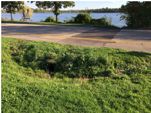
Figure 5.34. Storm Drain at VPD
