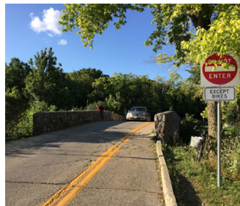
Figure 5.53. Stonework of Bridge
