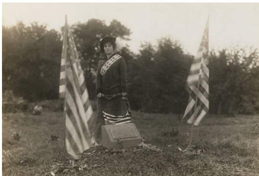
Figure 5.152. Tablet on Concrete Block, 1914 Wisconsin Historical Society - WHI-51985
