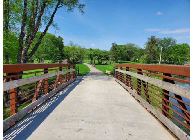
Figure 5.56. Bridge Concrete Surfacing
