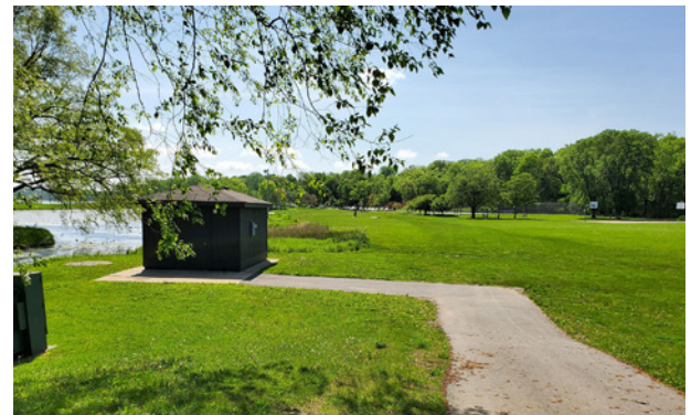
Figure 5.12. Pump House in Summer
