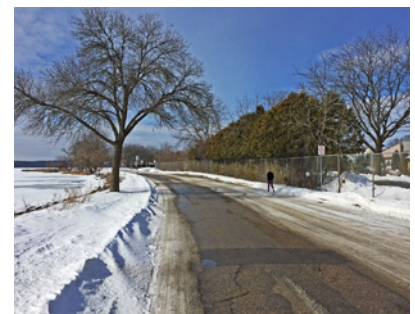
Figure 5.78. Corridor in Winter
