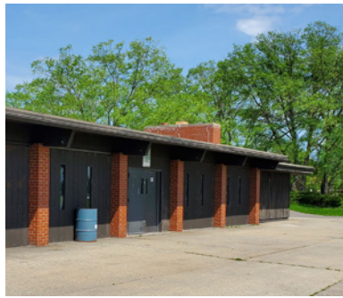
Figure 5.2. Shelter Tuck Pointing
