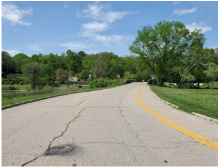
Figure 5.31. Longitudinal Cracks
