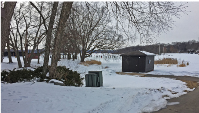
Figure 5.11. Pump House in Winter
