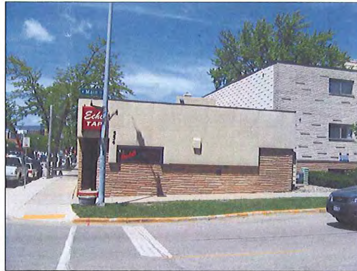
EXISTING MAIN STREET FACADE
