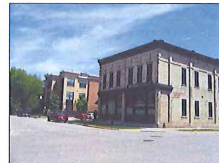
EXISTING STRUCTURE IN NEIGHBORHOOD
