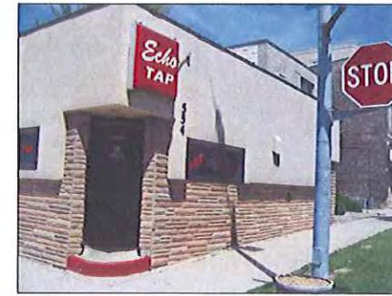
EXISTING FRONT ENTRYWAY
