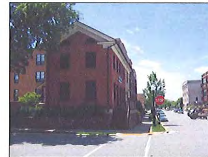
EXISTING STRUCTURE IN NEIGHBORHOOD
