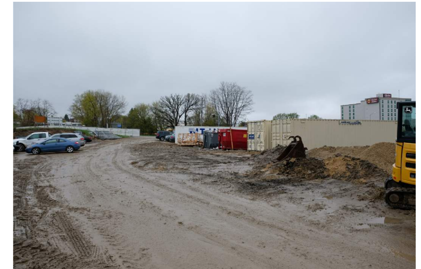
SOUTHEAST CORNER OF LOT LOOKING NORTHWEST
