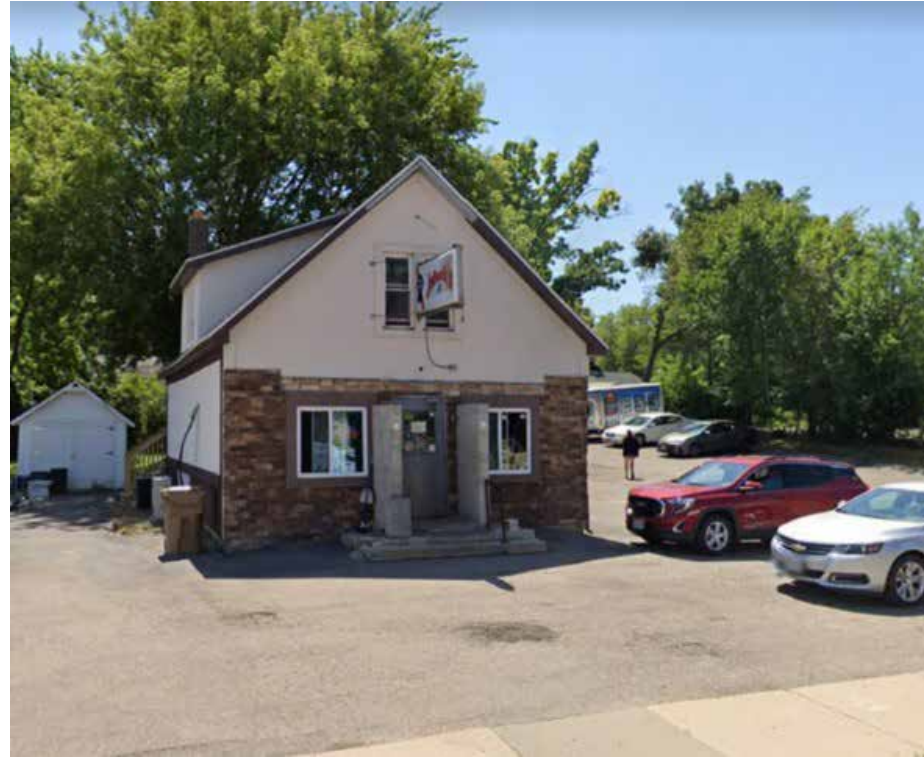
#105 521 Cottage Grove Rd (The Dive Inn) Not completed
